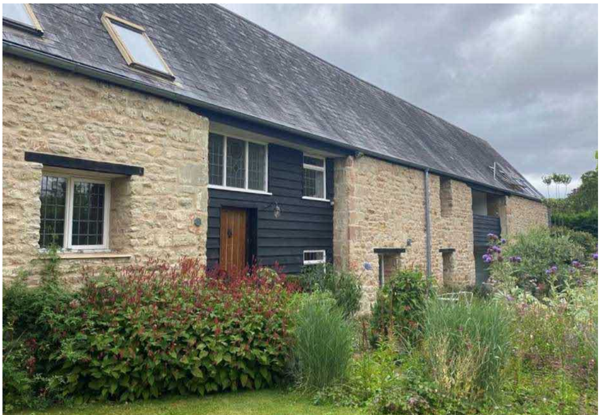
Figure 8 Barn Western frontage from the garden
