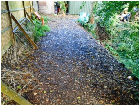
Figure 3 View of the northern end of the site. Note: the cutting was back filled when the original bridge was removed.
