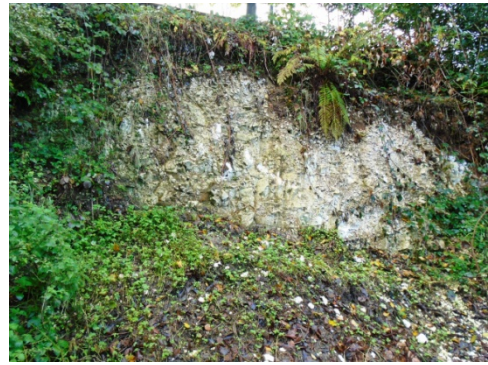
Figure 7 View of part of the chalk face on the south western side of the cutting.
