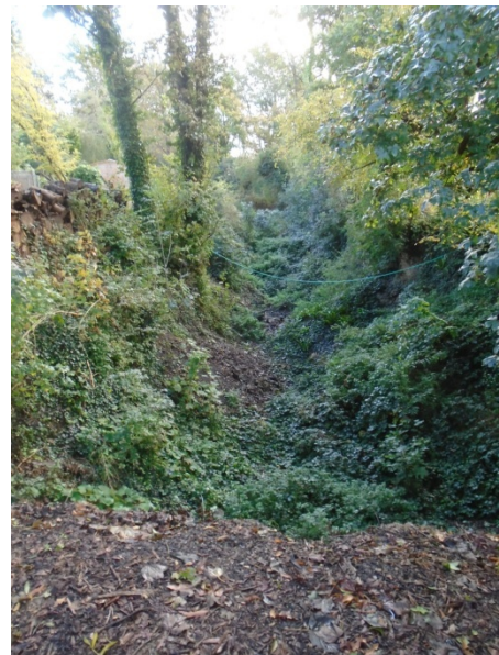
Figure 4 View looking south along the ditch, from the northern boundary.
