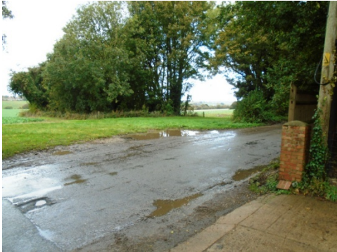
Figure 1 View looking north over Church Road, the line of trees denote where the cutting was.
