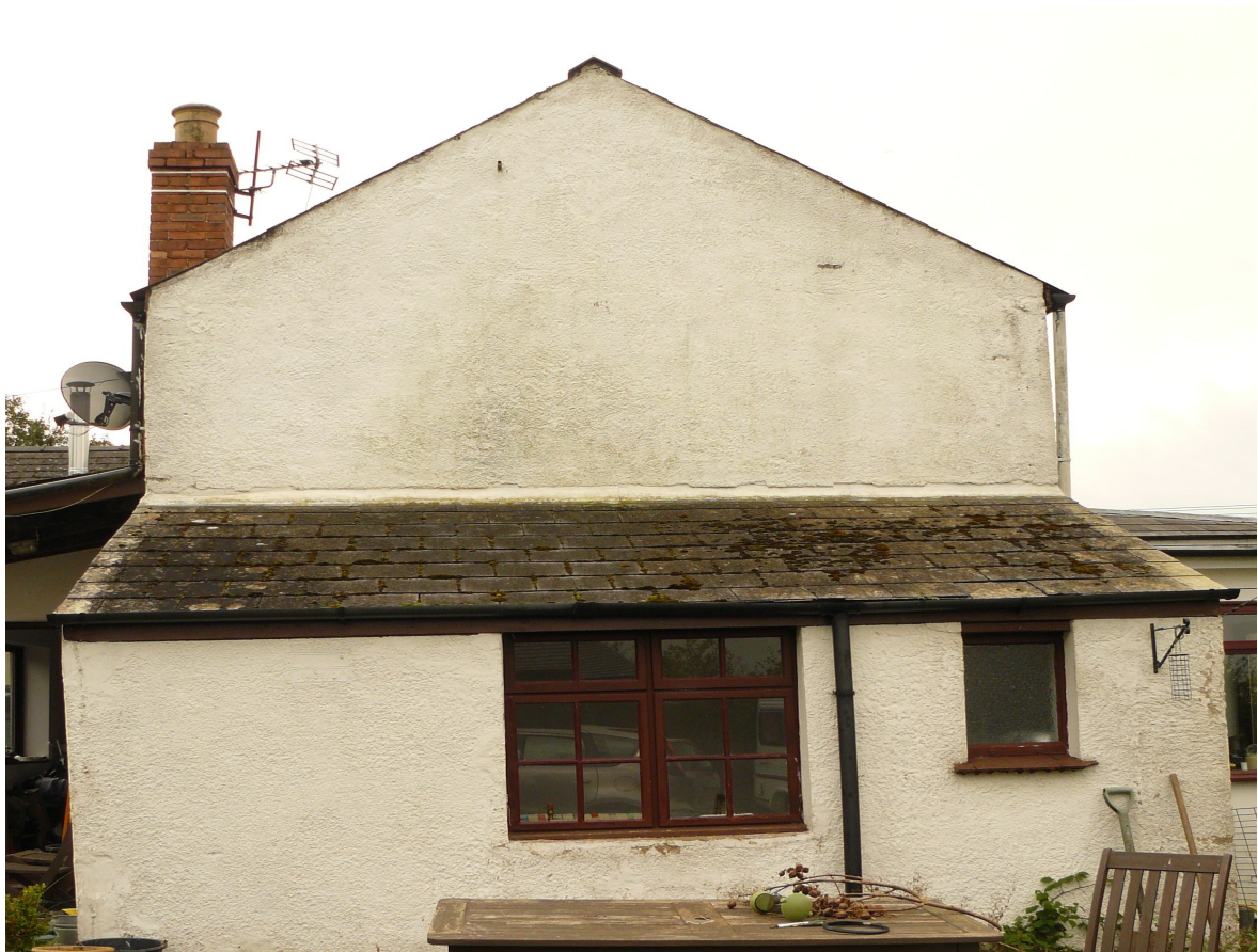
Picture 4: Lean-to and Gable End of Cottage
