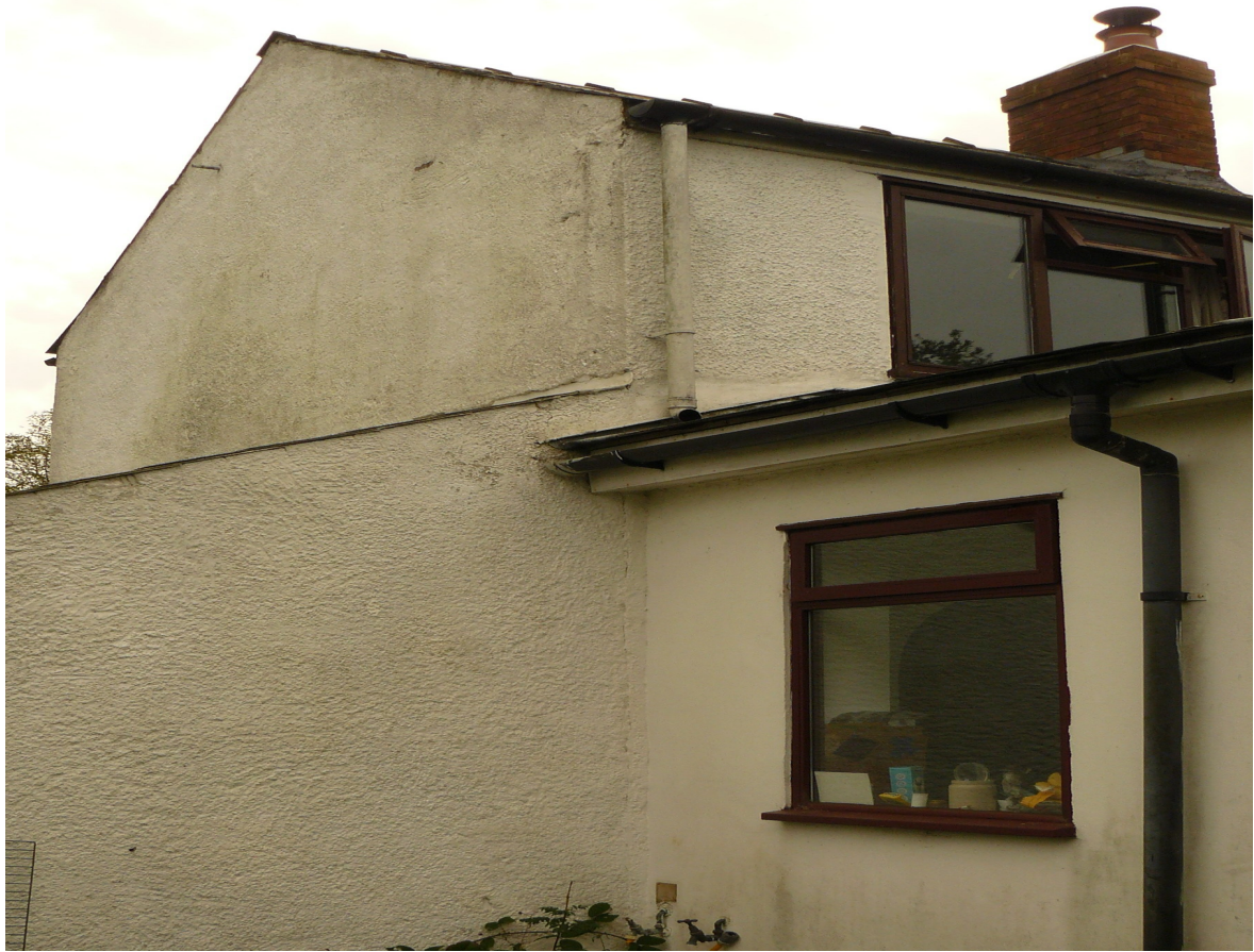
Picture 3: Corner of Lean-to, Gable End and Front Single Storey
