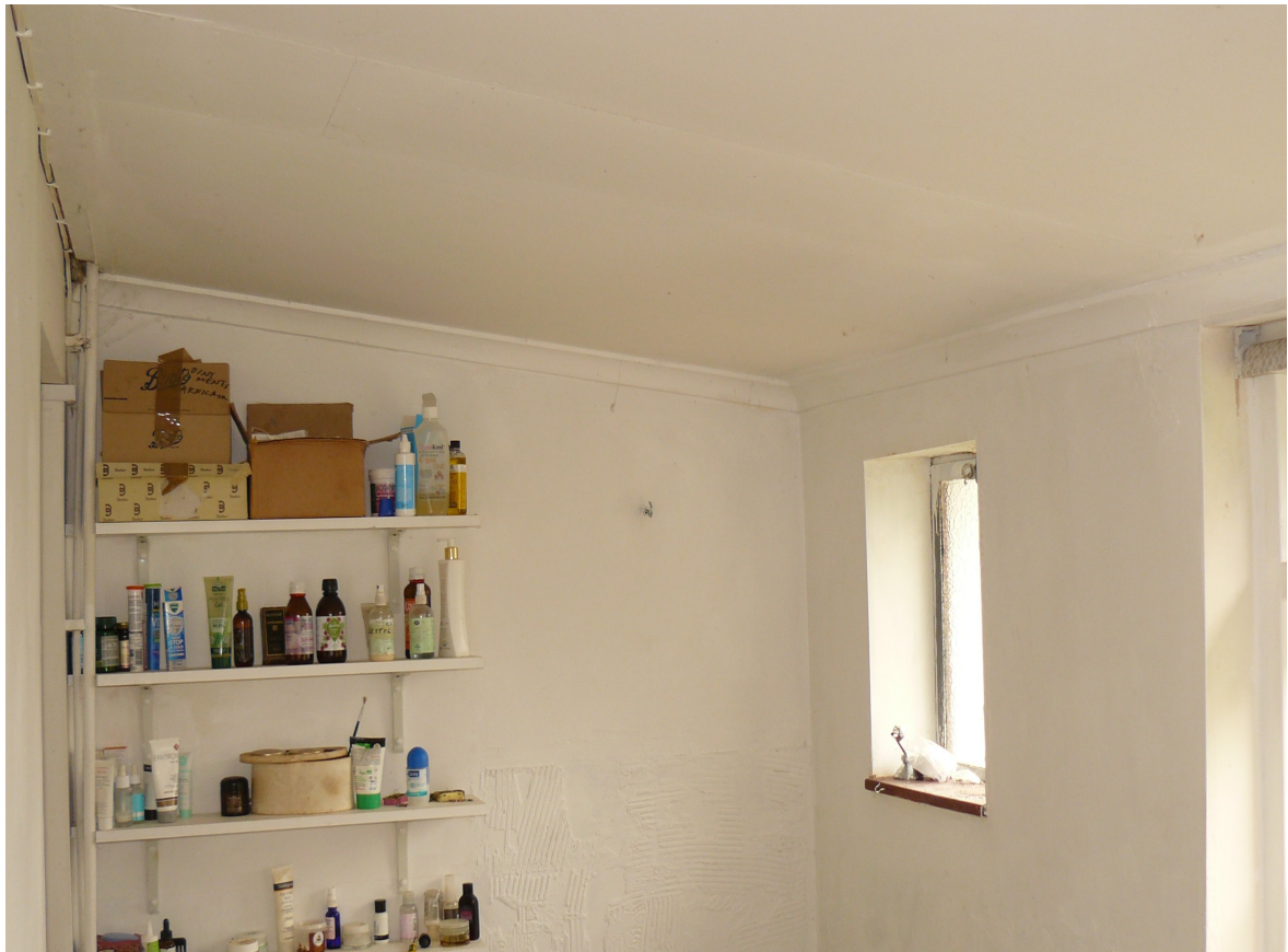
Picture 11: Interior of Lean-to (bathroom)
