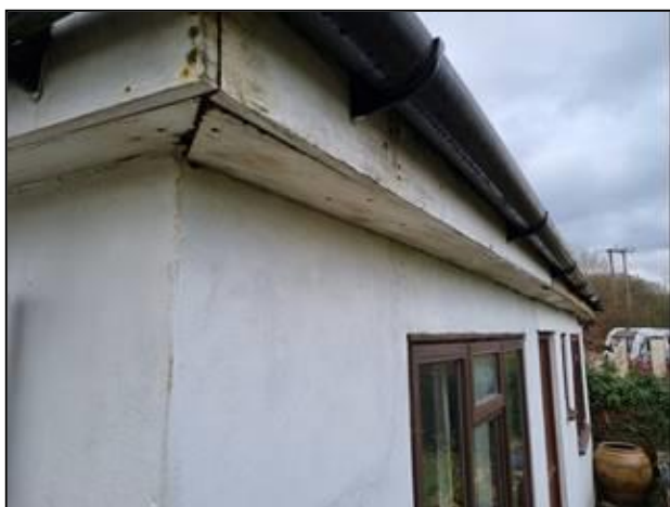
Photo 3 – Ground floor lean-to – sealed soffits
