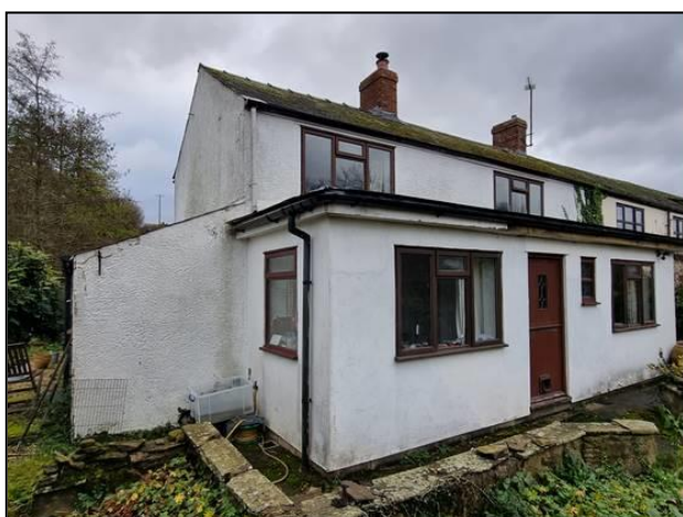
Photo 1 – General north-west elevation view
