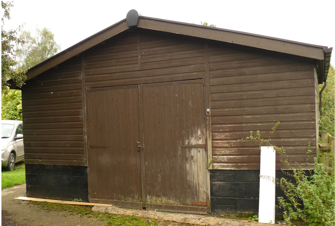
Picture 9: Side of Garage
