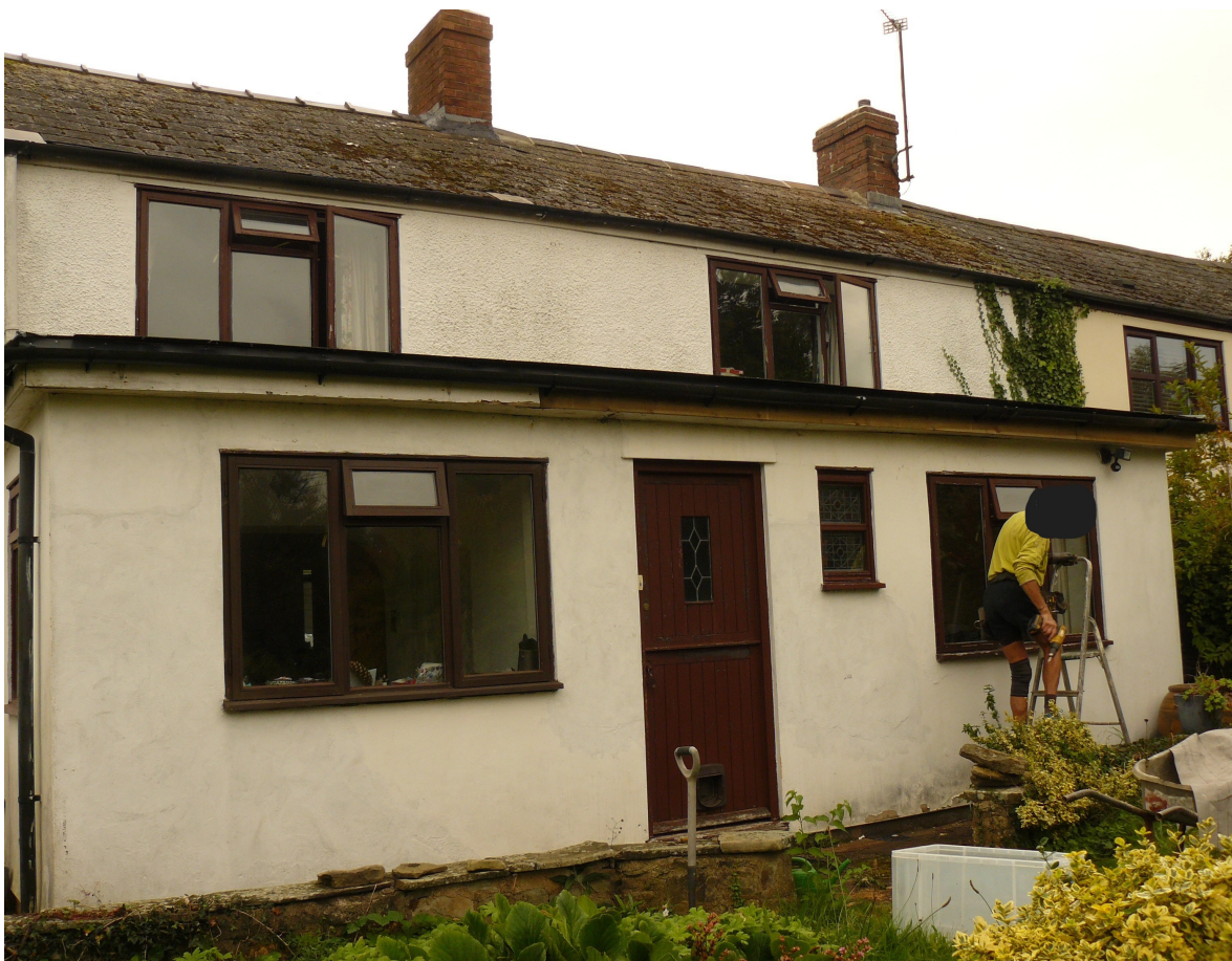
Picture 2: Builder Replacing Fascia Boards of Front Single Storey
