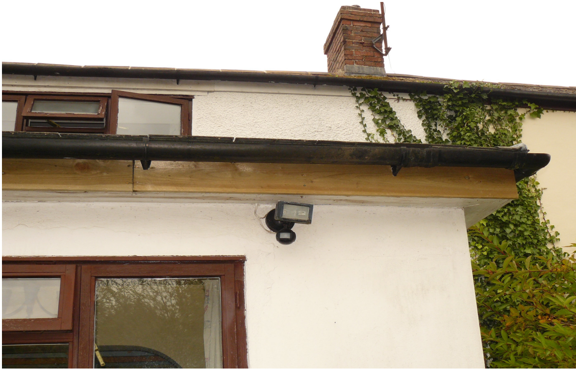
Picture 1: Eaves/Fascia of Front Single Storey
