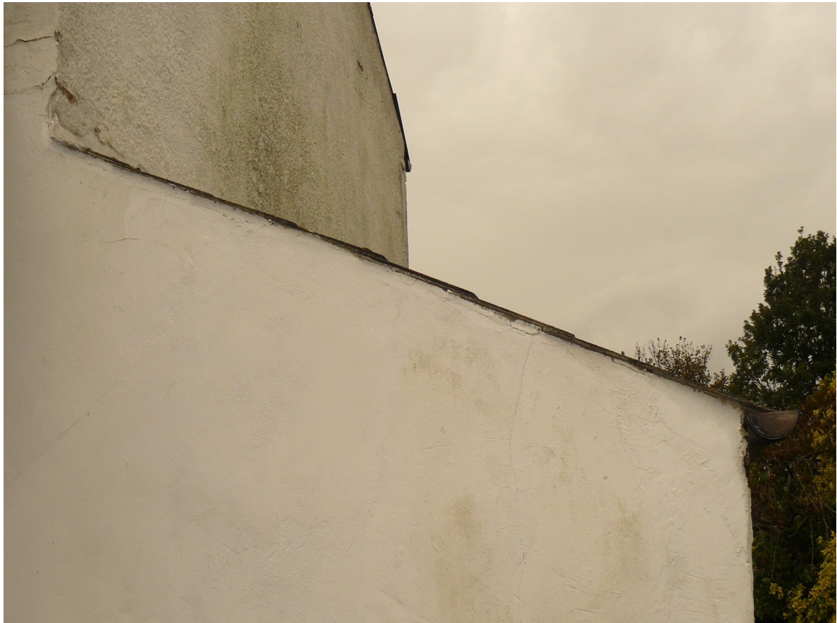
Picture 7: Side of Lean-to from Rear
