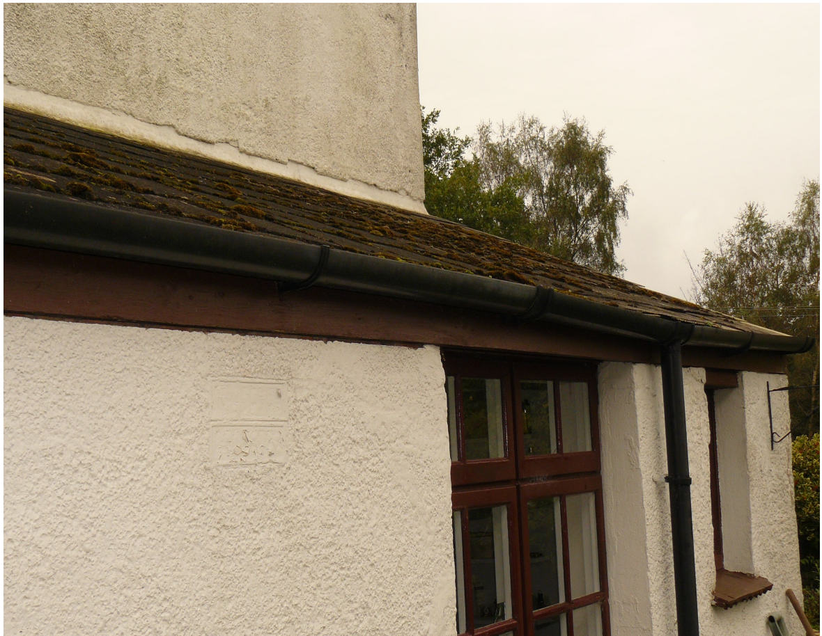
Picture 6: Fascia of Lean-to
