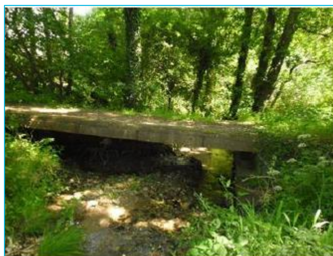
Figure 1-4: Footbridge, upstream of Forder/Bircham Stream confluence
