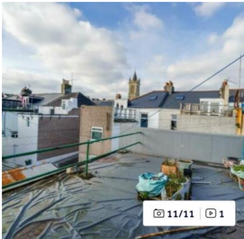
Below is a Google earth image from 2005. It can be seen on this image that the roof room and roof terrace are already in situ:
