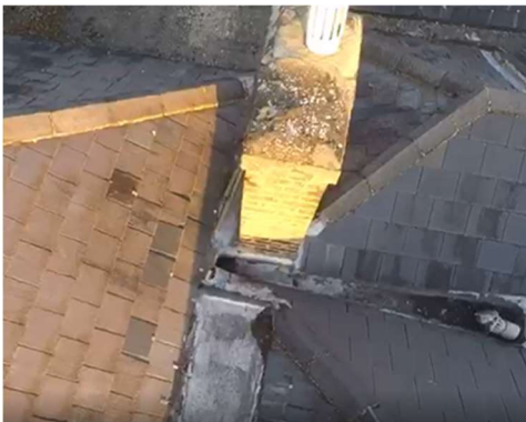
Roof outlet adjacent to chimney
