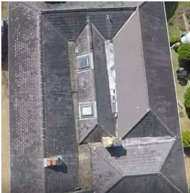
Roof form showing extended North end
