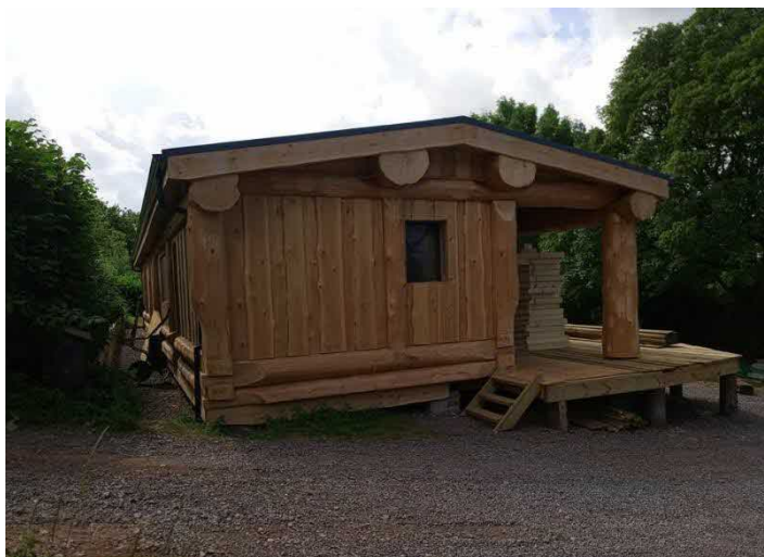
Figure 9: Example photos of similar cabins (Source: BLC)
