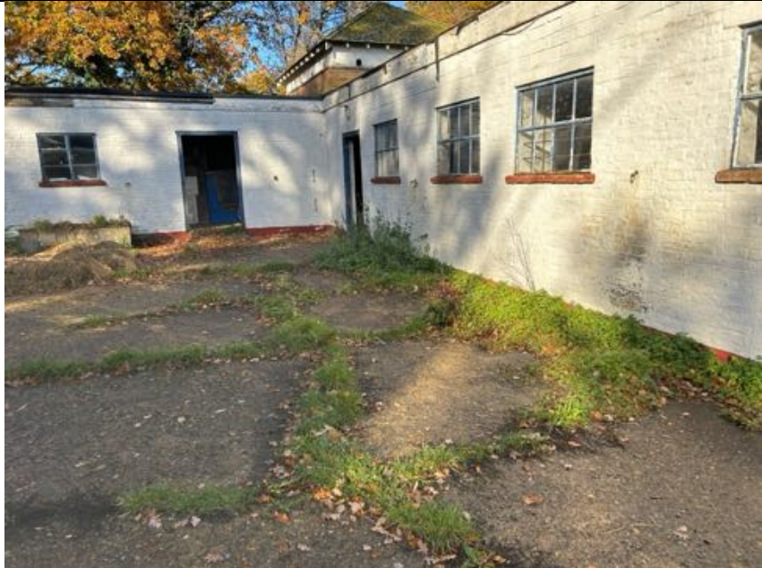
Photograph 6: Hardstanding in the centre of site
