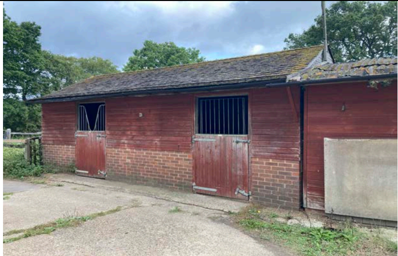
Photo 1: The stables to the north east (B1)
