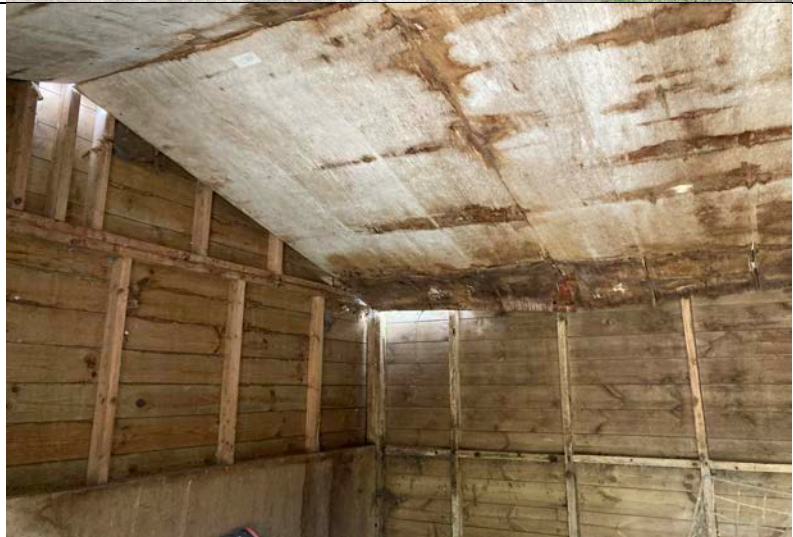
Photo 2: Internal stables to the north east.(B1)
