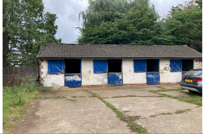
Photo 5: The stables to the south west of the site (B4)
