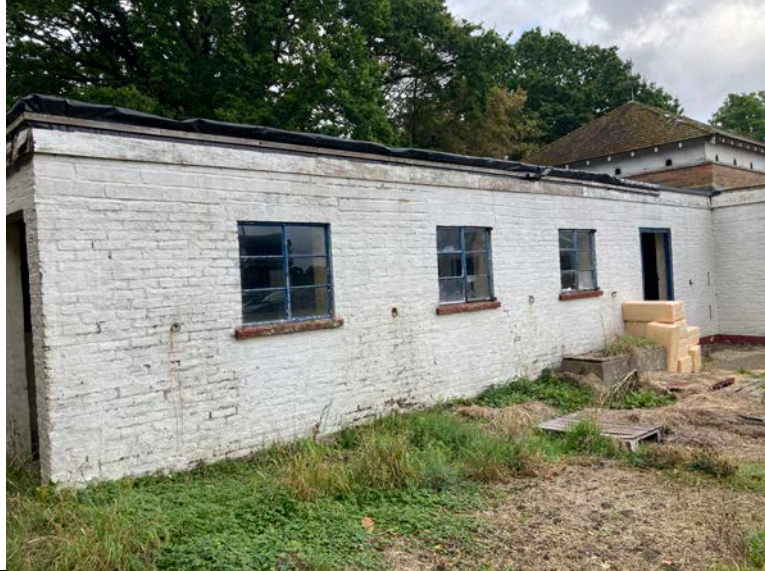
Photo 7: Buildings B5 on the western side of the site.
