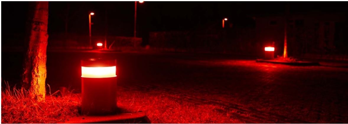
Figure 7: Example of low level bollard lighting
