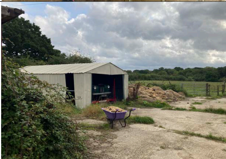
Photo 3: The metal barn (B2)
