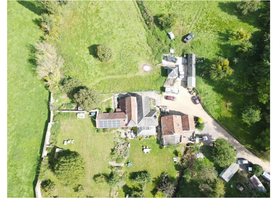
Image Above | Existing site
