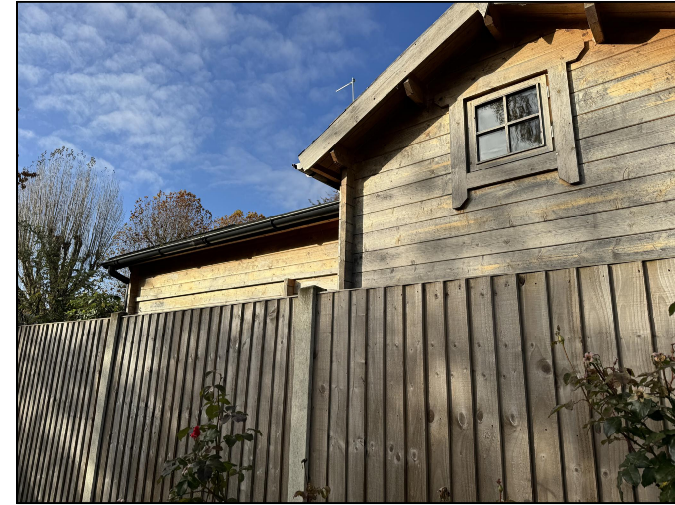
Photograph showing outbuilding on adjacent land to North-West boundary
