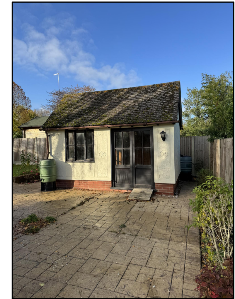
Photograph showing front elevation of existing outbuilding
