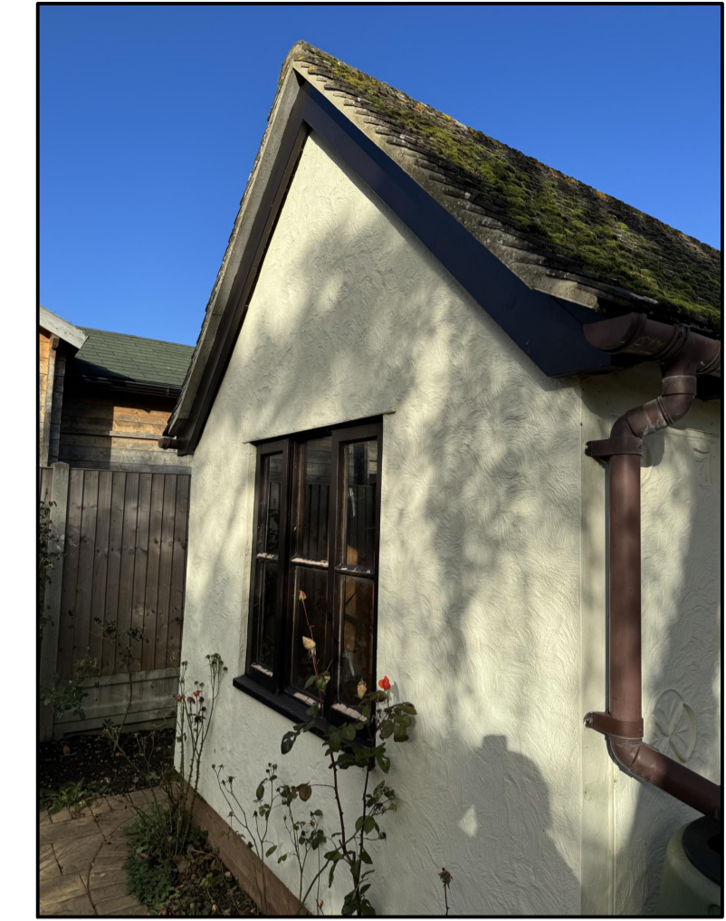
Photograph showing side elevation of existing outbuilding
