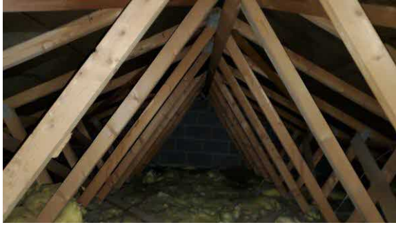
9 internal view of loft
