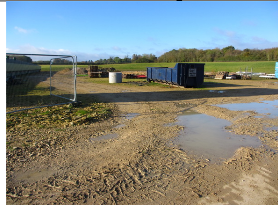
Photo 1: North-west view of the site
