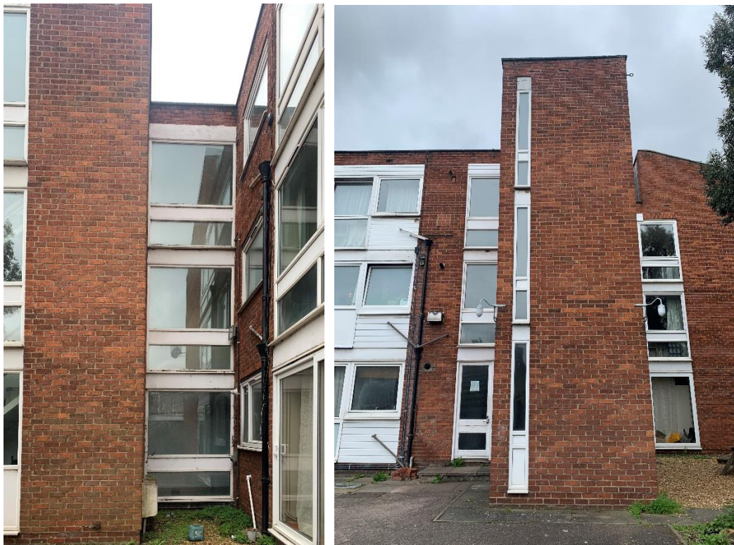
Photograph of location for new lift behind existing stair enclosure
