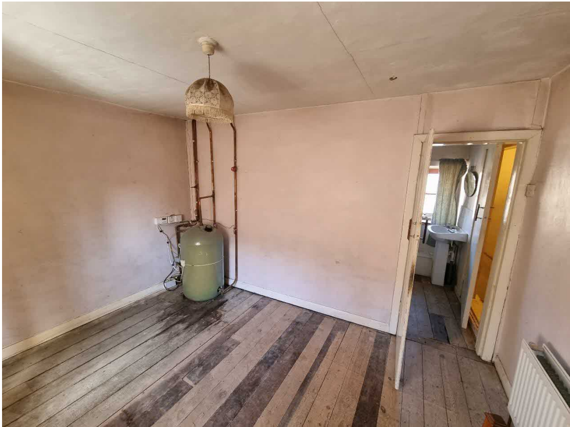
Photograph No. 14 – View On To Front Bedroom/Bathroom Dividing Wall
