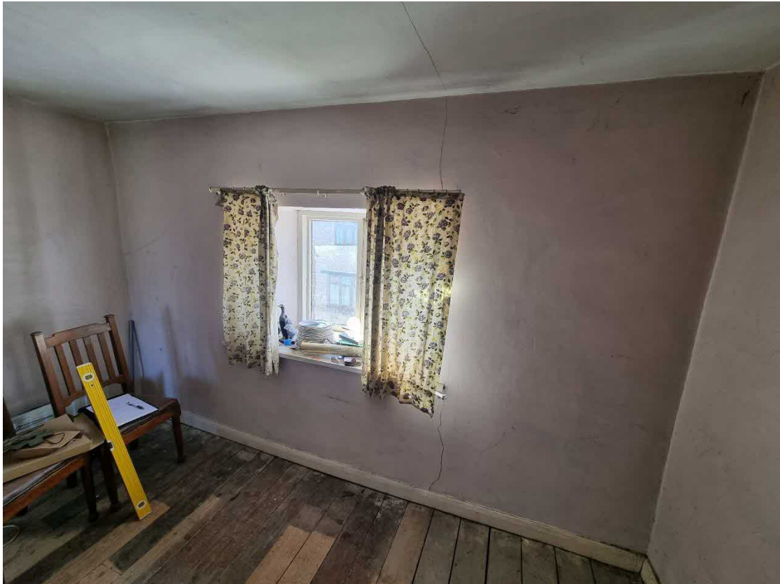
Photograph No. 13 – View On To Front Wall Of Front Bedroom
