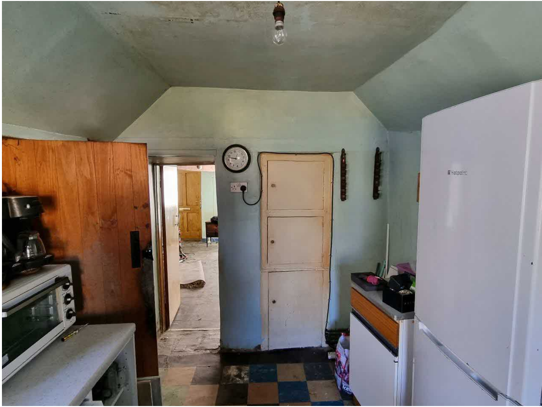
Photograph No. 7 – View On To Lounge/Kitchen Dividing Wall From Kitchen Annex
