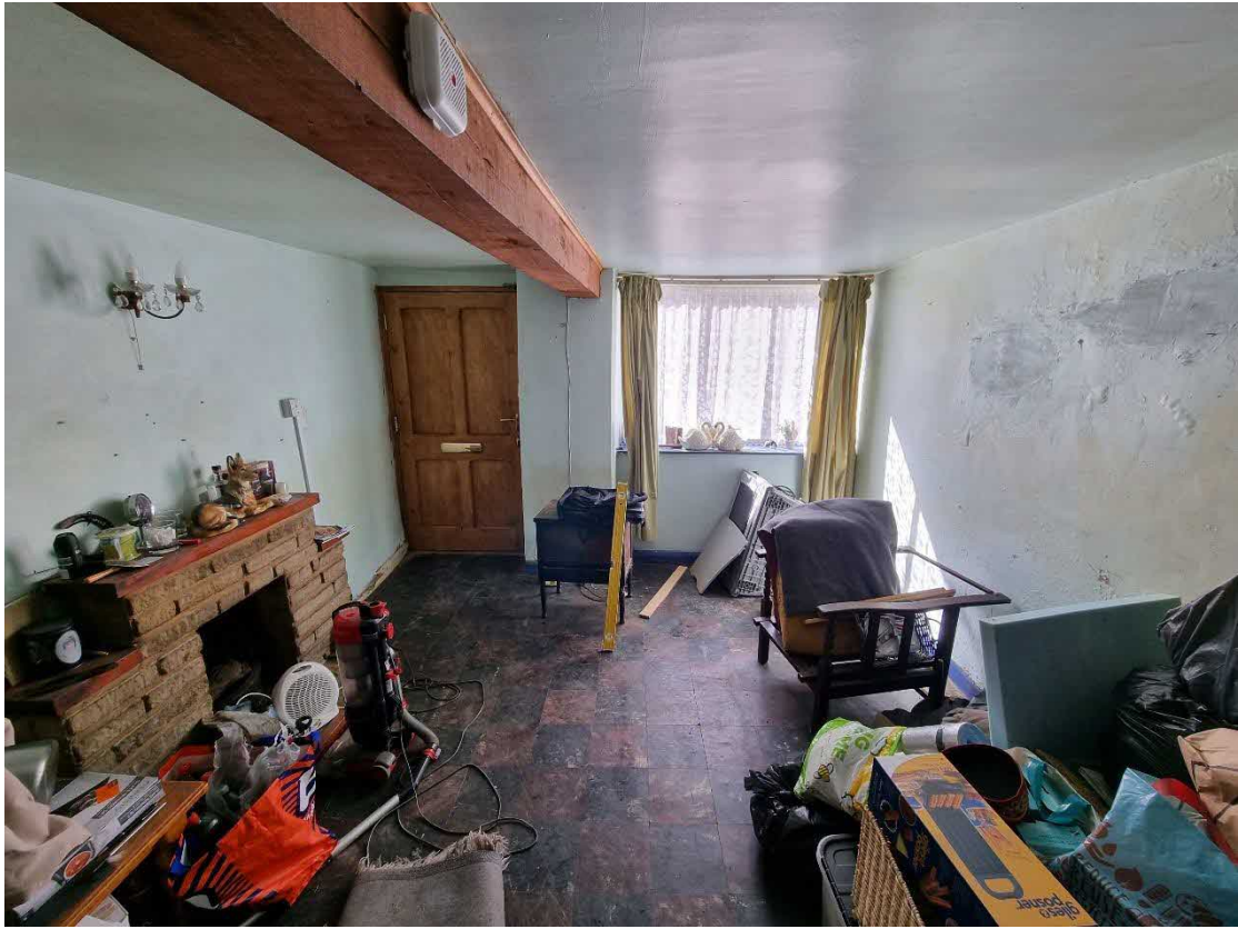
Photograph No. 5 – Internal View From Kitchen Annex Toward Lounge Front Wall
