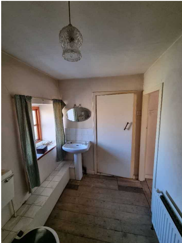
Photograph No. 16 – View On To Bathroom/Stairwell Dividing Wall
