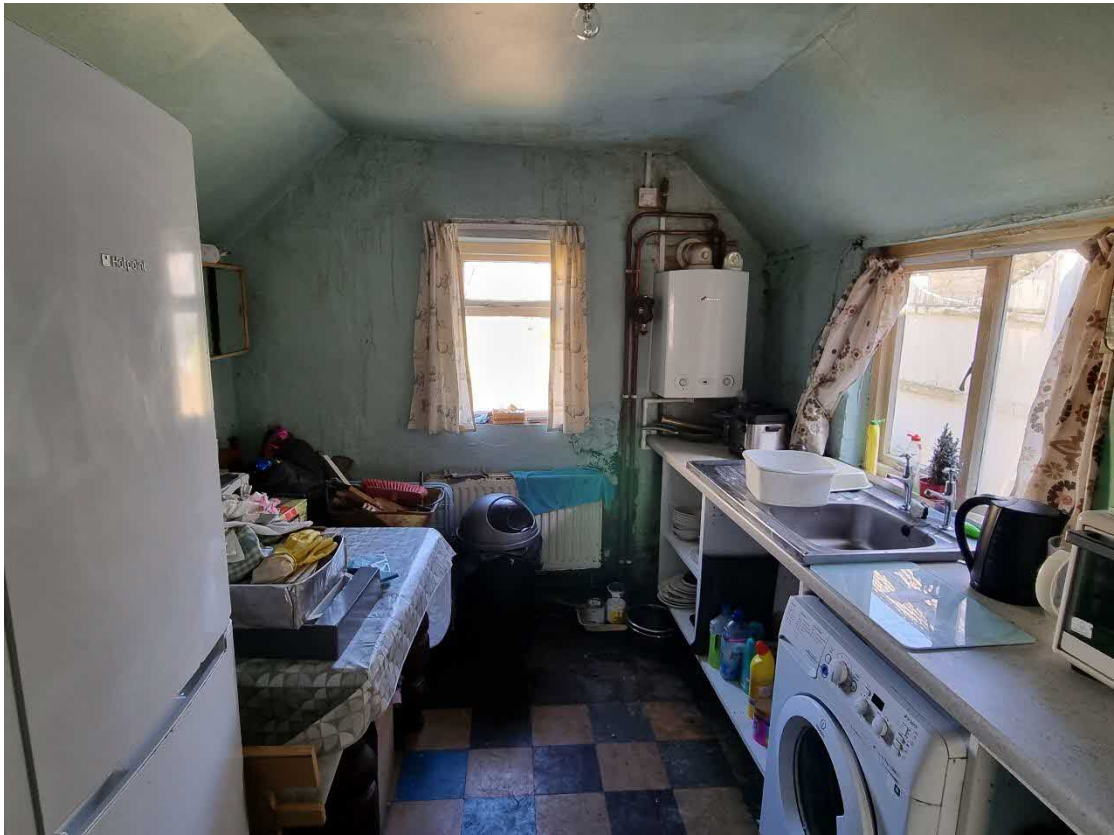
Photograph No. 6 – Kitchen Annex Rear Wall
