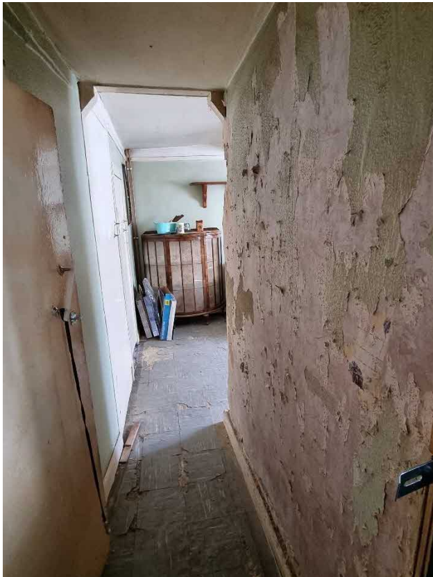
Photograph No. 8 – Corridor From Lounge To Ground Floor Right Hand Bedroom
