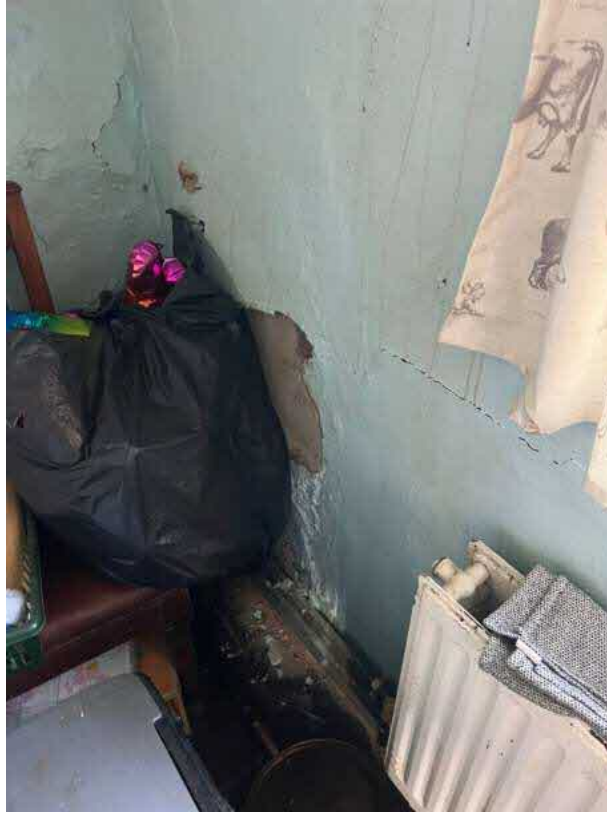
Existing kitchen walls current condition.
