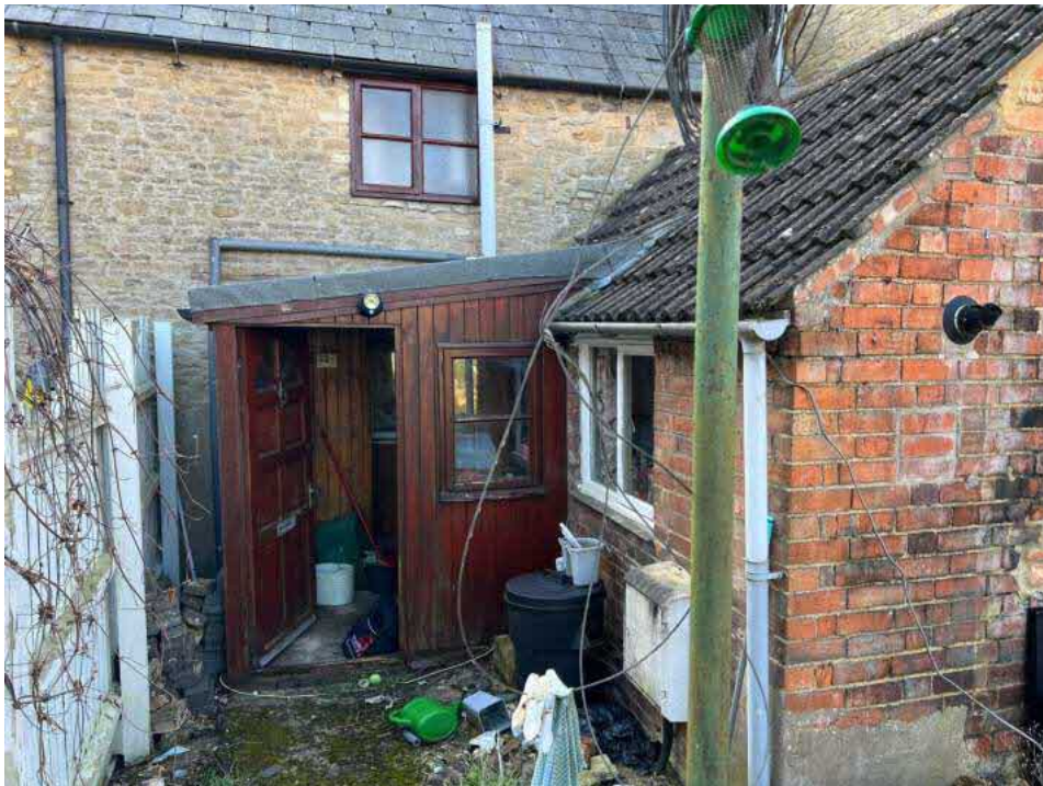
Existing ground floor leanto timber structure
