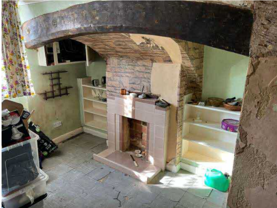
Fire place and feature curved beam to be retained.
