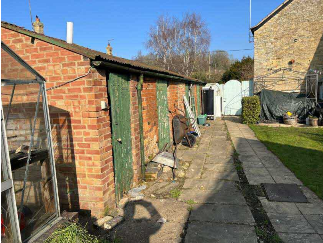
Existing garden outbuildings
