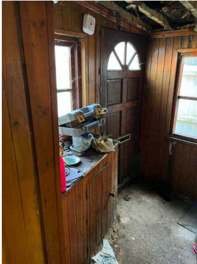
Existing ground floor leanto timber structure.
