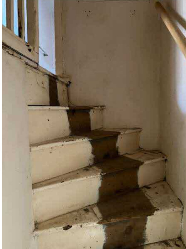
Existing staircase top of flight
