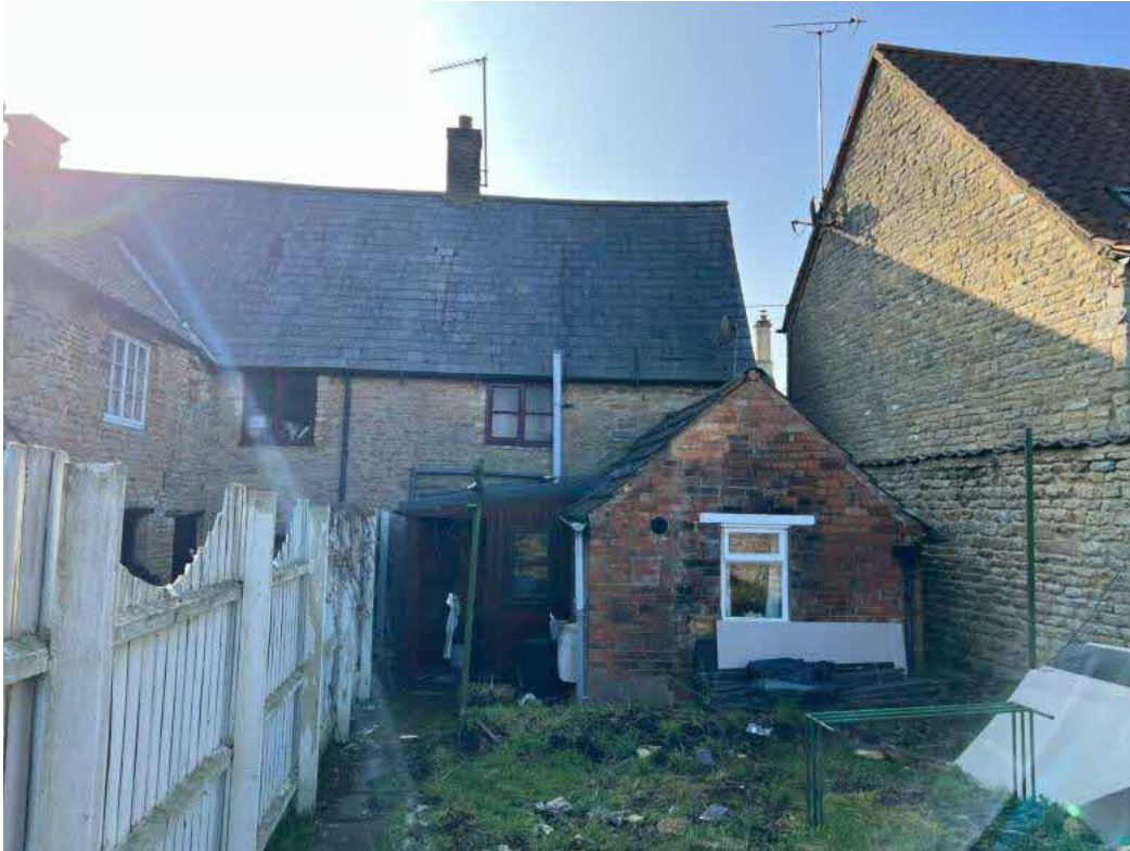
Existing rear elevation showing stone wall, brick and timber extensions.
