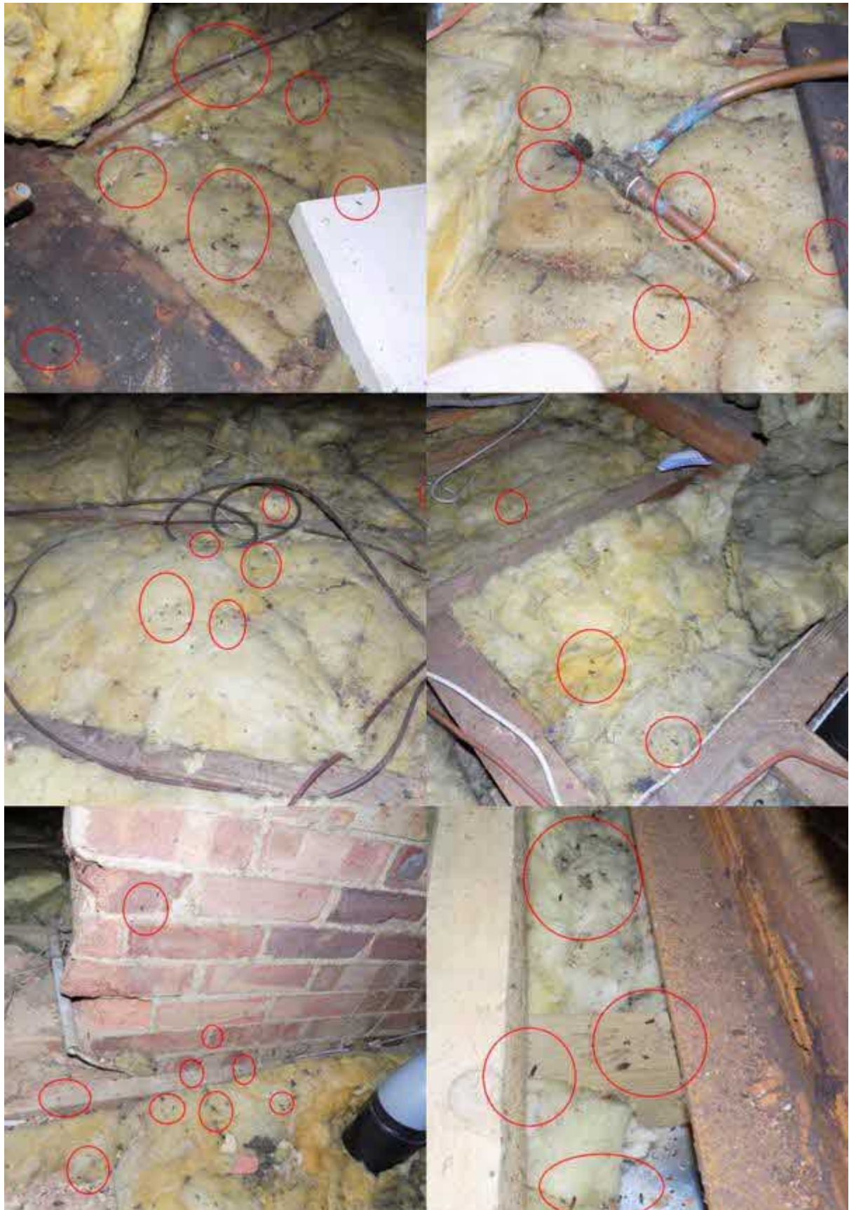
Image 8 – Activity from bats within the form of bat droppings across multiple areas of the roof void spaces with dense piles below sections of the ridge
