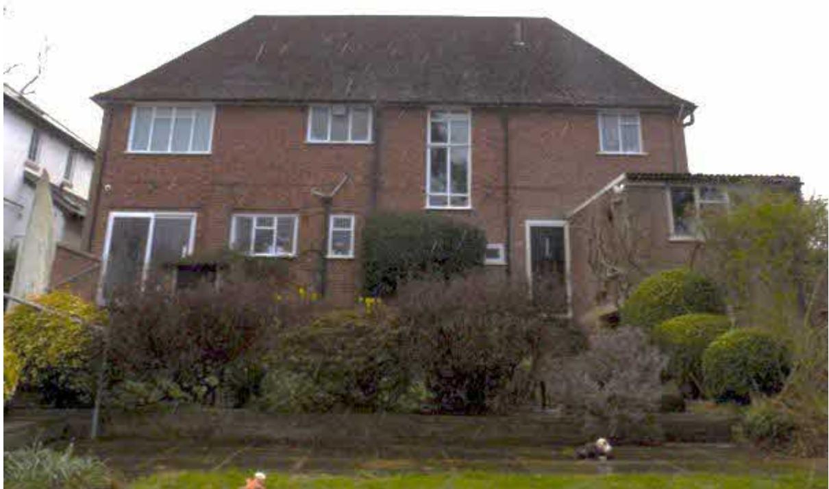
Image 3 – North facing elevation of the property
