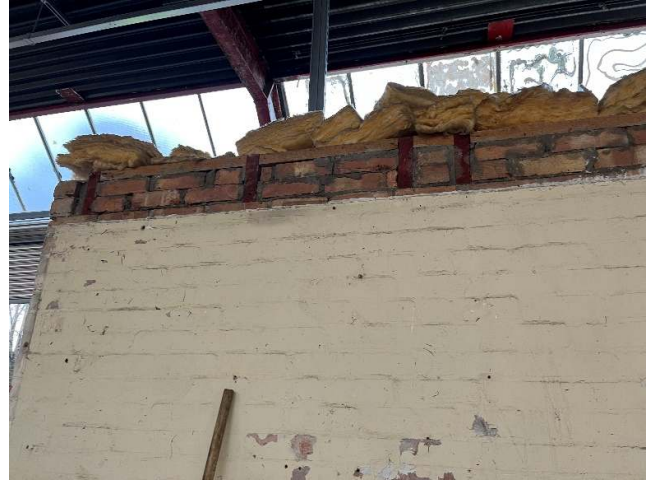
Photo 10: Internal wall surrounding welfare facilities
