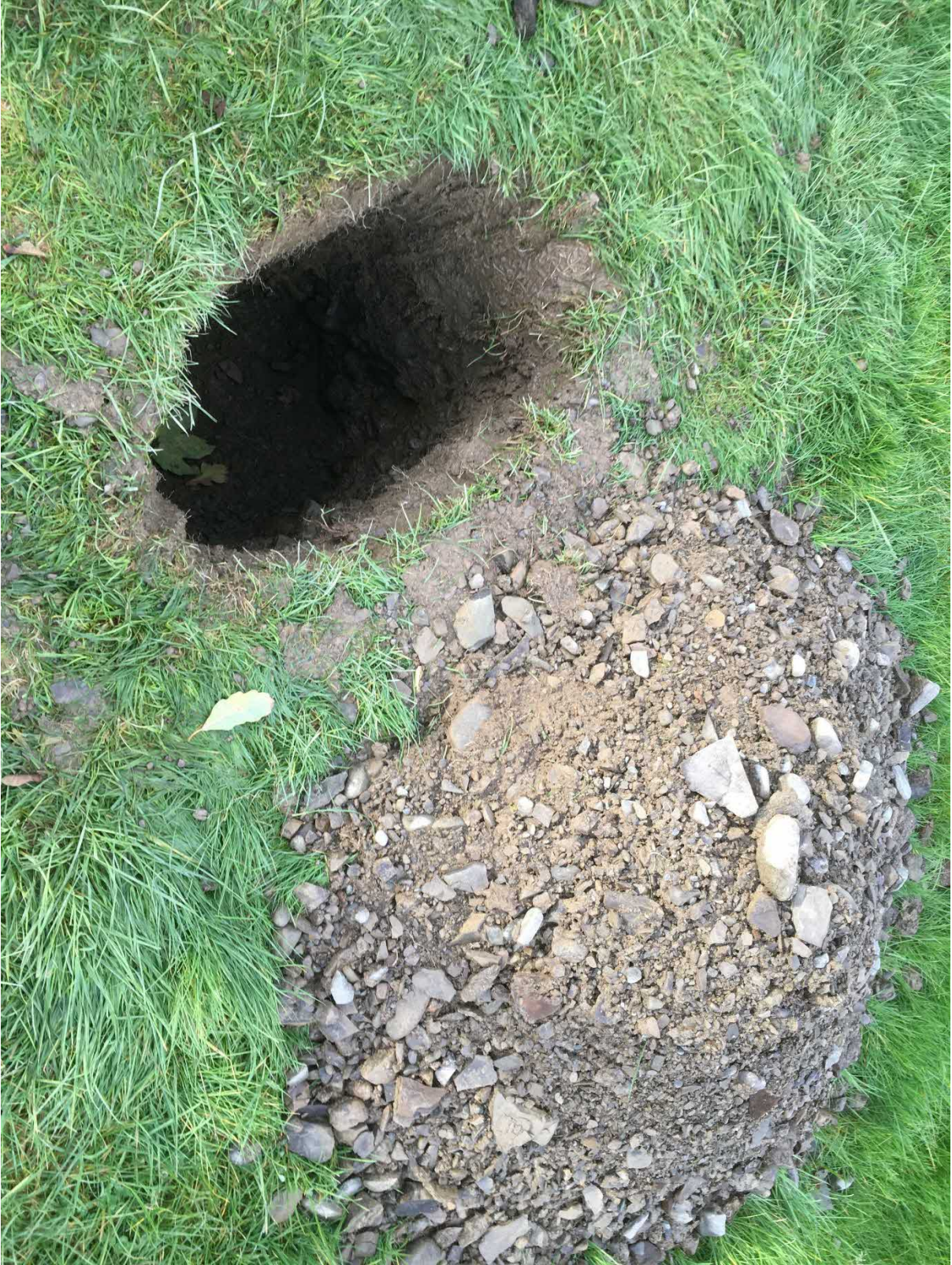
Image of test hole/excavated material.
