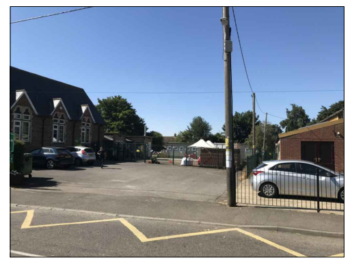
Survey photo of the school from the street existing mobile at the rear of the site
