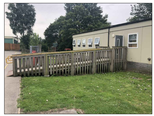
Survey photo of the existing mobile Ramp
