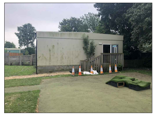
Survey photo of the existing mobile RH side elevation
