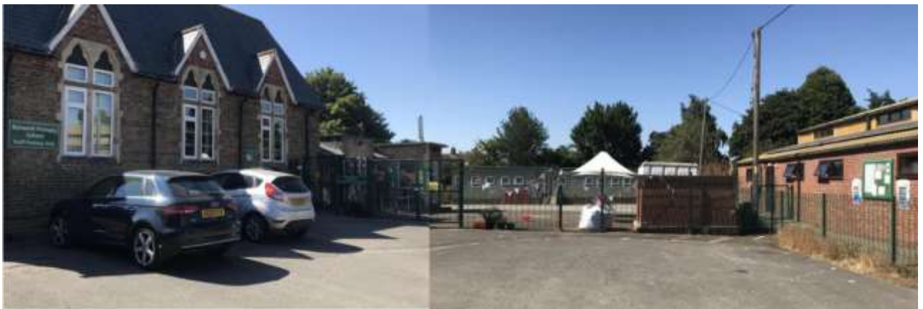
Main School frontage with the existing mobile classrooms in the distance behind the playground, with the school car parking in the foreground between the school buildings and village hall
