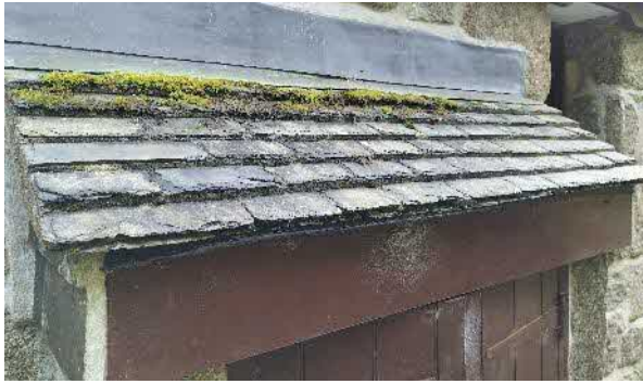
Figure 5. The small, sloped roof on the northern extent.
