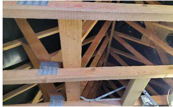
Figure 6. The roof void of the garage
