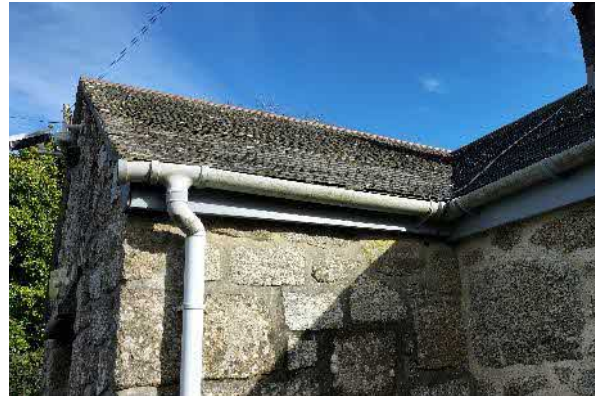
Figure 2. The building viewed from the south
