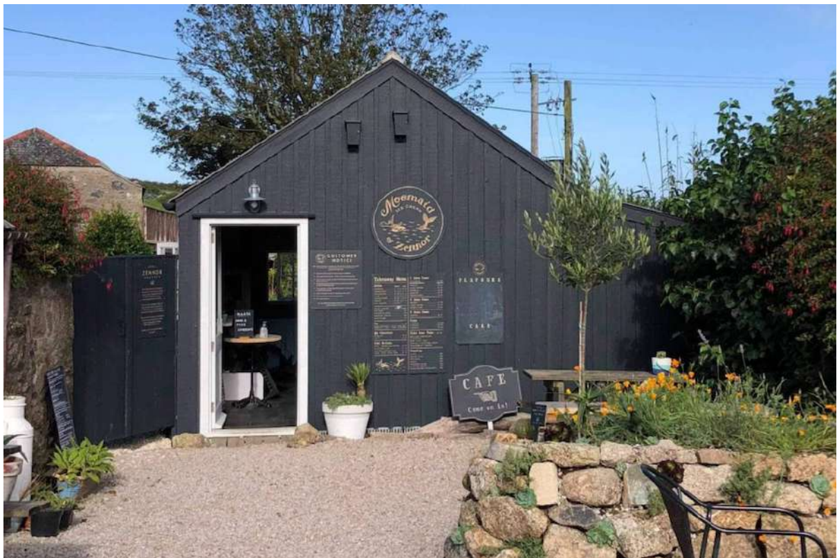
Moomaids of Zennor Ice Cream Parlour, example of vertical timber board and batten cladding.
