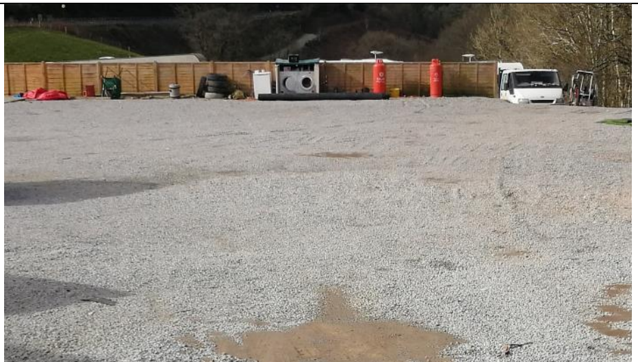
Photo 6: Showing the feather-board fencing present across some areas of hardstanding.
