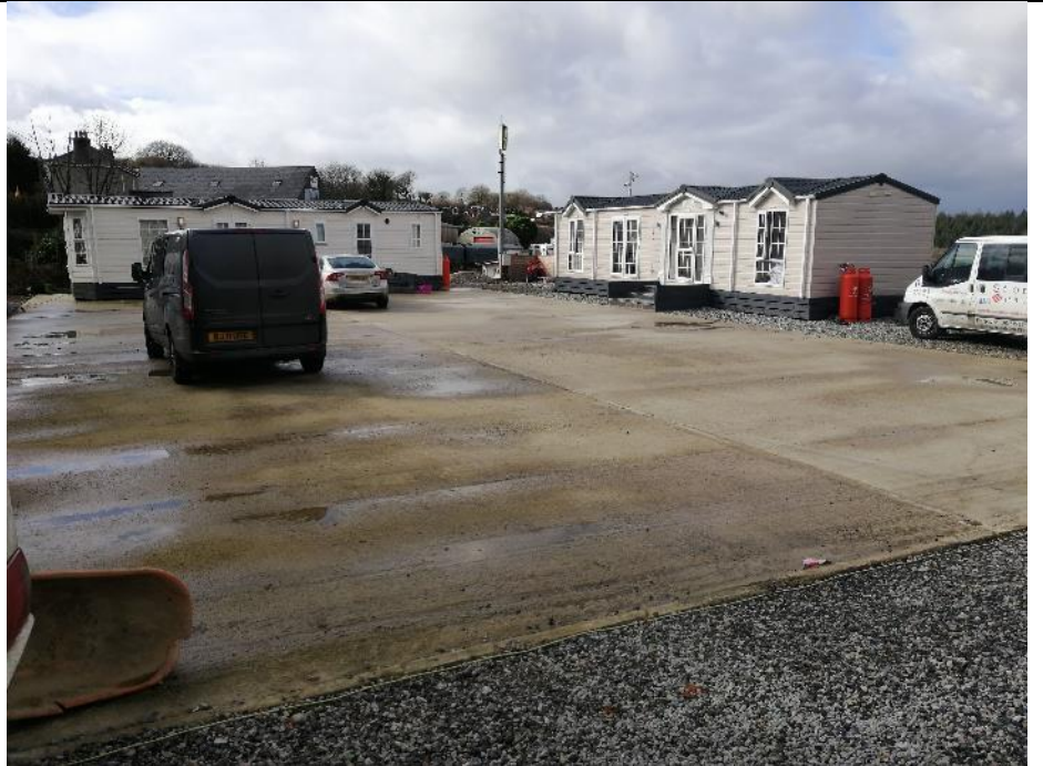
Photo 7: View of the mobile homes situated on the concreted area of hardstanding.
