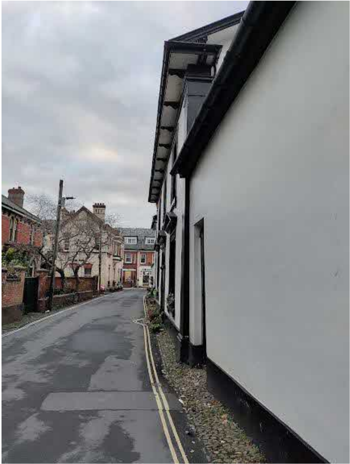
Figure 5 -Side view of property façade on Church Street
