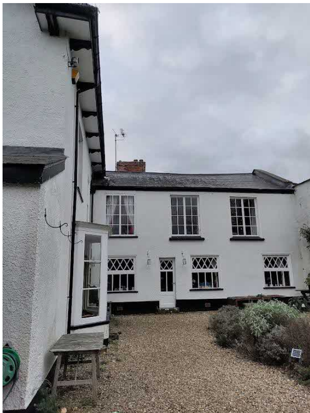
Figure 7 – View of rear extension (unaffected by the proposals)
