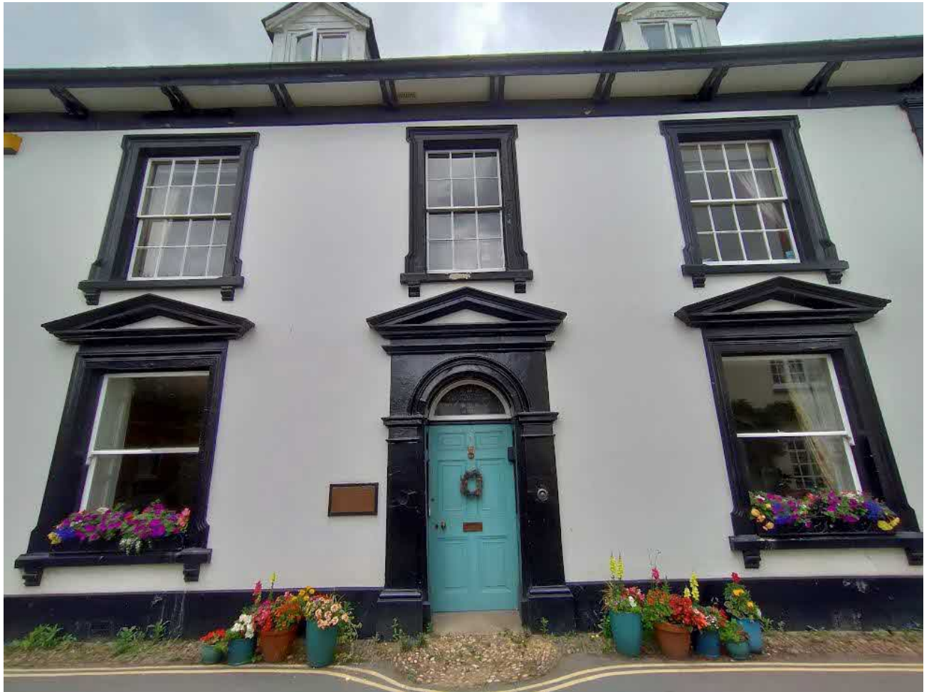
Figure 4- Front elevation, showing original windows on First Floor and later windows on Ground Floor and Second Floor/attic
