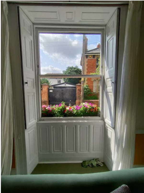
Figure 8 –Sitting Room window (Ground Floor)
