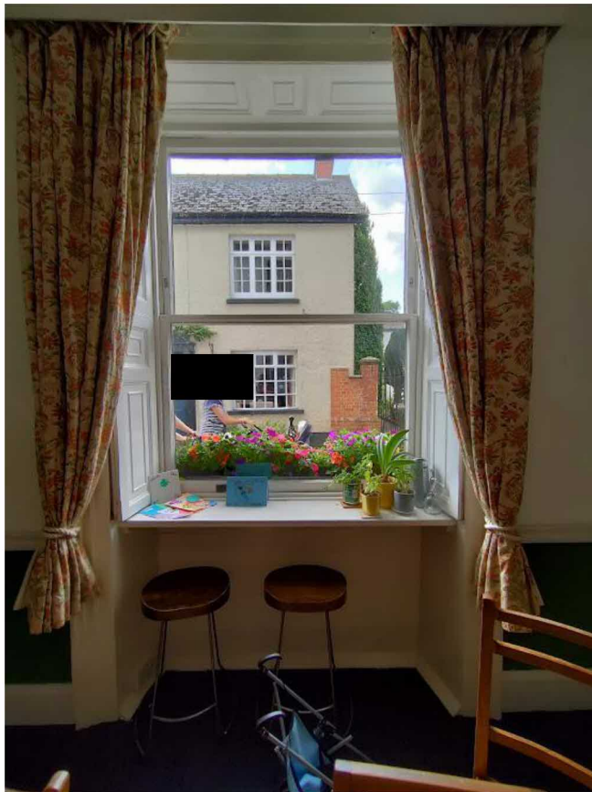
Figure 9- Dining Room window (Ground Floor)
