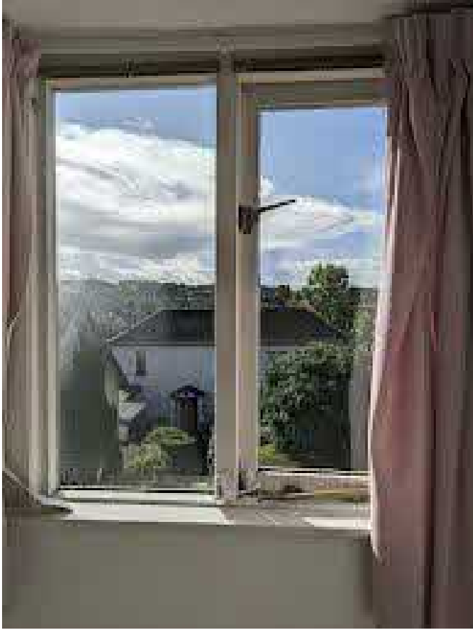
Figure 12 – Bedroom 5 window (Second Floor/Attic)
