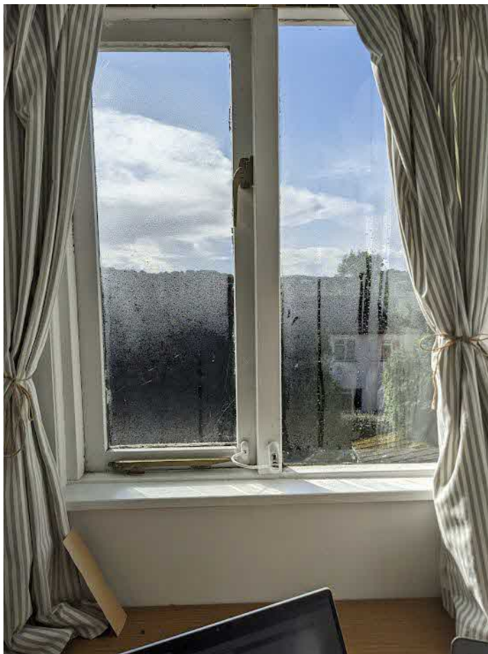
Figure 11 - Bedroom 4 window (Second Floor/Attic)
