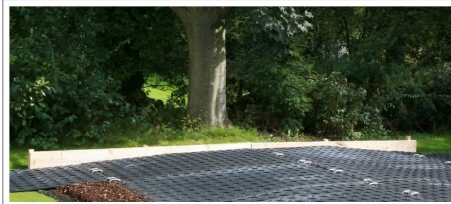
Figure 2: Example of temporary ground protection boards
