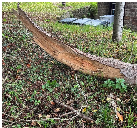
Image 3: The recently failed east facing limb with no visible decay at the point of failure.
