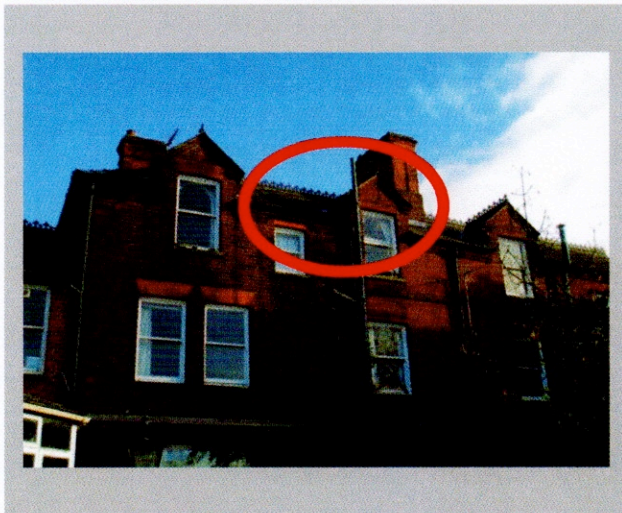
Photograph 3: Roost 2, a common pipistrelle day roost (1 x bat) in an area of missing mortar and damaged brickwork and guttering at eaves level on the western elevation of a section of B1 to be demolished.
