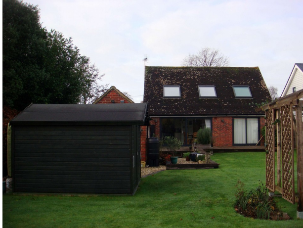
House rear/east and shed
