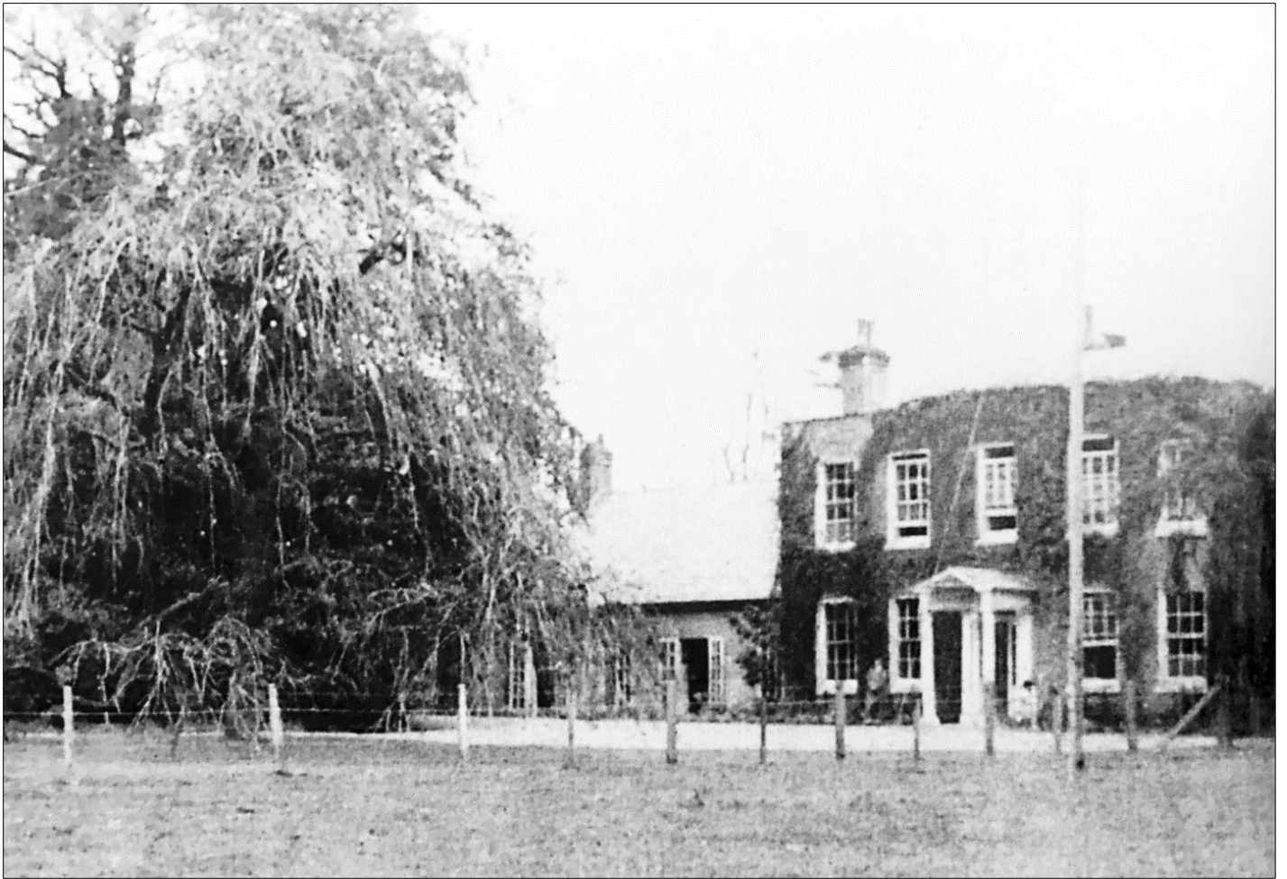
Fig. 27 Stonar House in the 1920s, looking east
