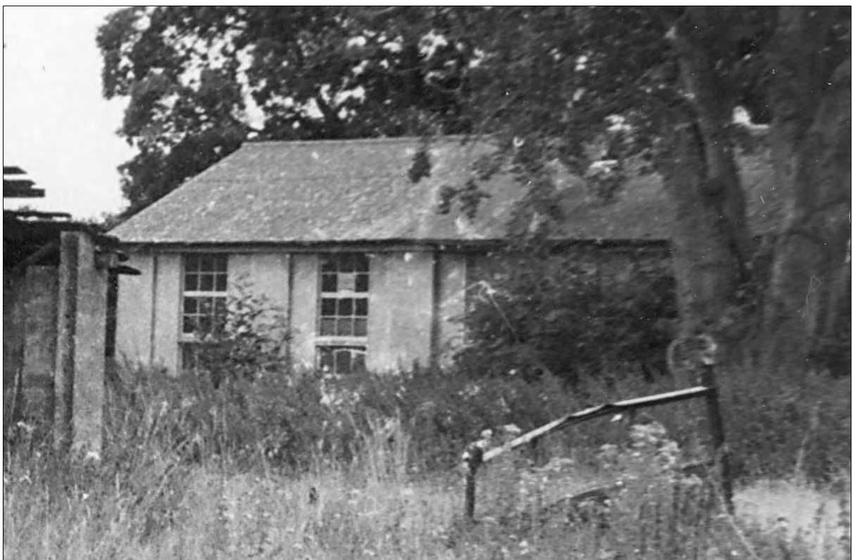
Fig. 40 The north end of the former Regimental Institute, looking north-east
