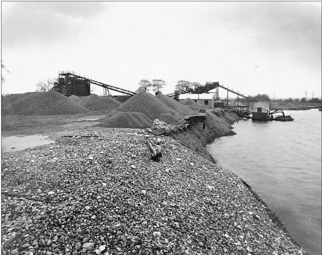
Fig. 64 The stock piles, looking west, mid-1950s
