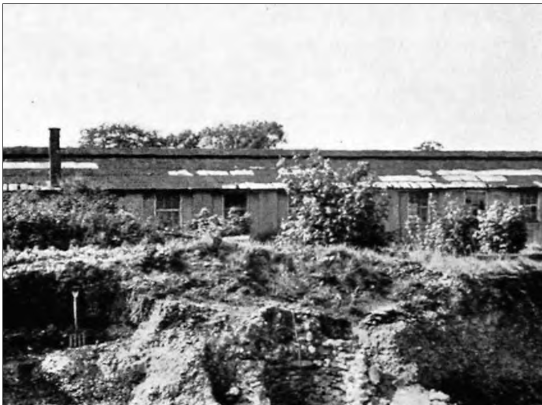
Fig. 57 The southern edge of the North Lake advancing on Building 64 during the late 1930s (archaeological excavations in foreground)
