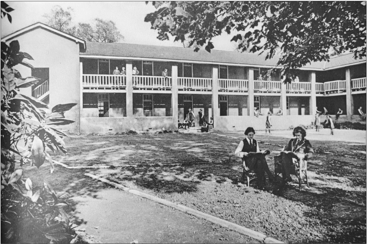
Fig. 49 The quadrangle, looking north-east
