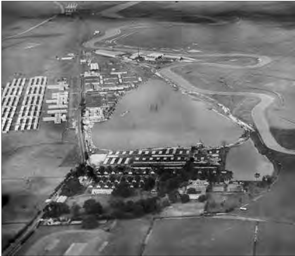
Fig. 54 Stonar Camp in 1927, looking north before much demolition had taken place (©Britain from Above; EPW018589)
