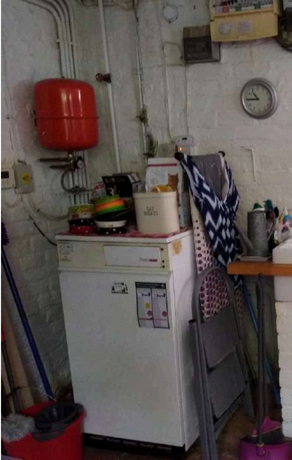
6. The White House existing boiler and dining room doors interior views
