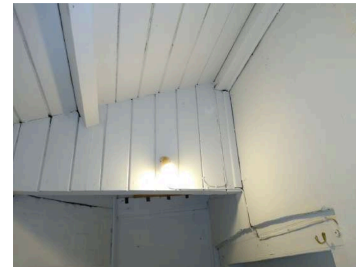
11. Lobby high level view
