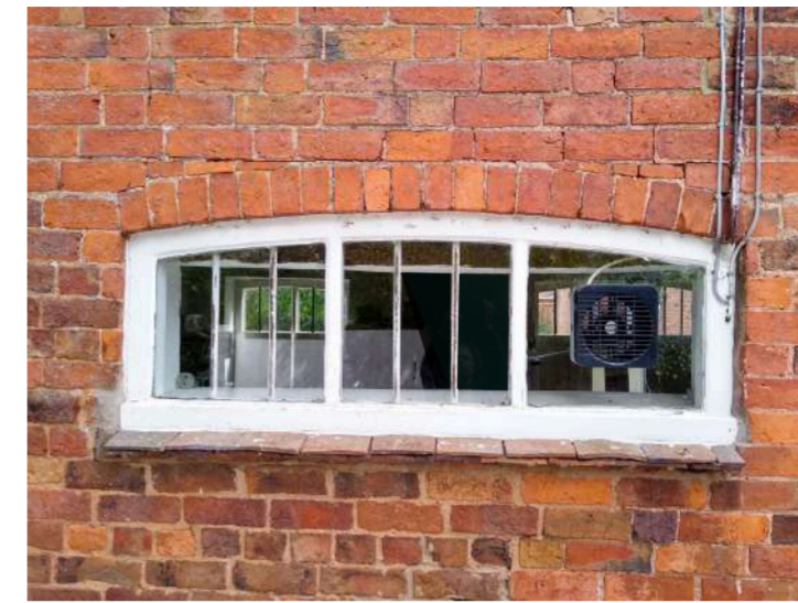
5. Utility Room W1 exterior of high level west window
