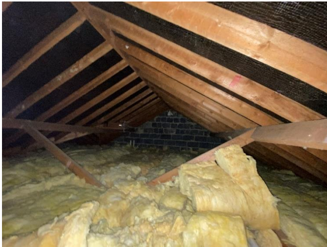
Photo 85: Roof space above the main property
