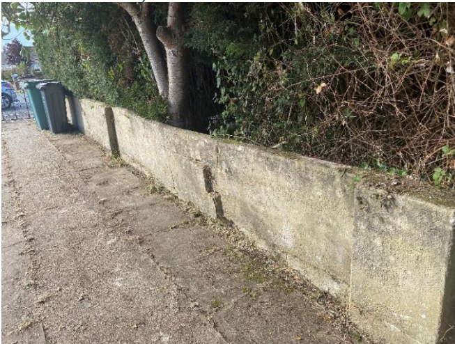
Photo 49: Cracking and movement to the boundary wall to the left hand side of the property. Damage at location of Cherry tree
