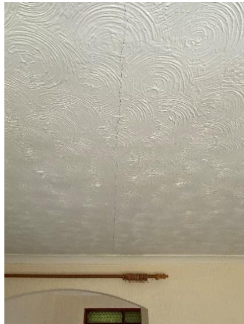
Photo 62: Cracking to the Front Reception Room ceiling
