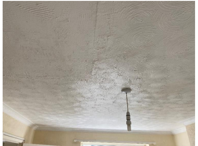
Photo 62: Cracking to the Front Reception Room ceiling
