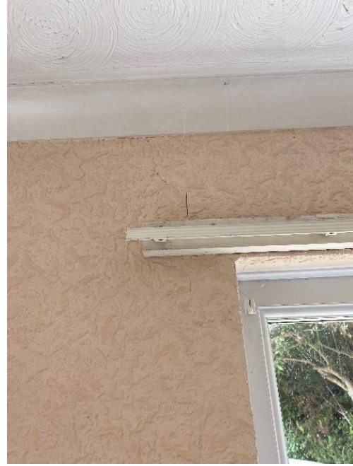
Photo 54: Isolated diagonal crack above the East side of the window to the front elevation of the Front Bedroom
