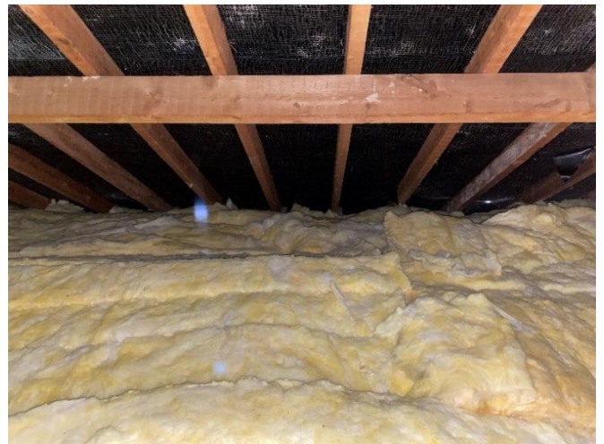
Photo 90: Raking struts to the East side of the roof space are not opposite or acting against each other
