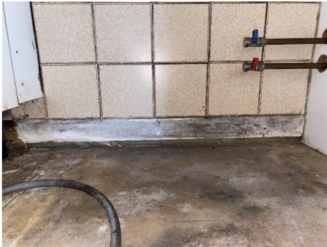
Photo 81: Gap between the underside of the skirting board to the rear external wall and the Kitchen floor below
