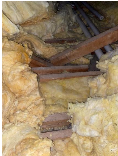
Photo 90: Raking struts to the East side of the roof space are not opposite or acting against each other
