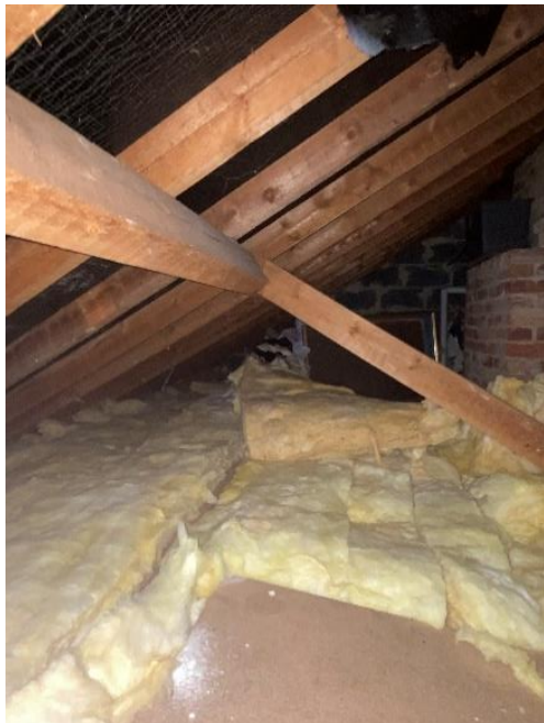
Photo 87: Roof space above the main property
