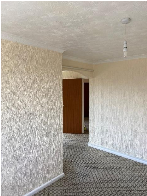
Photo 67: Opening within the wall which separates the Reception Rooms
