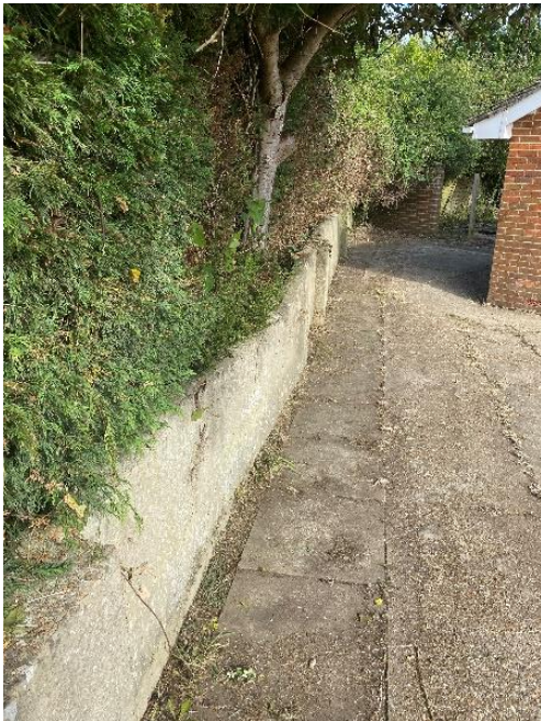
Photo 49: Cracking and movement to the boundary wall to the left hand side of the property. Damage at location of Cherry tree
