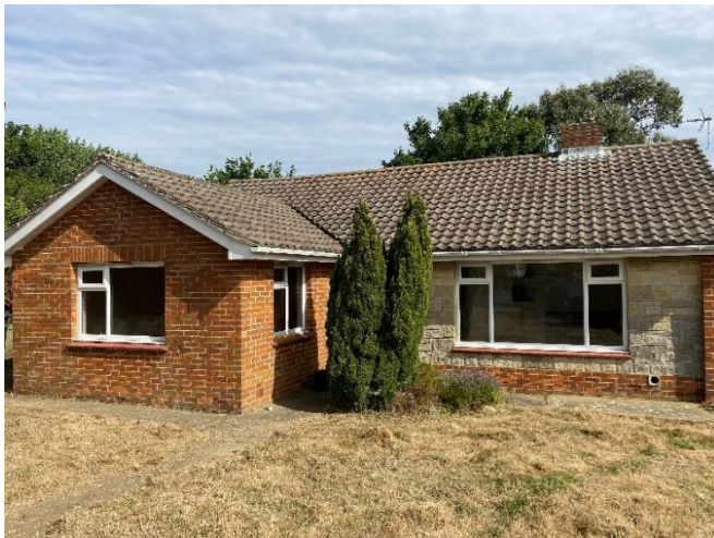
Photo 47: Conifer adjacent to the front right hand corner of the front projection
