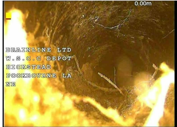
Sec_9_Insp_1_UnknownX_654.jpg, 00:00:03, 0.10 m Roots, fine
