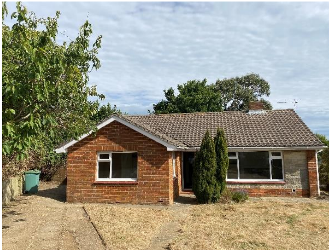
Photo 1: Front elevation of the property
