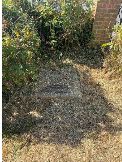
Photo 38: Inspection chamber to the South East corner of the front garden
