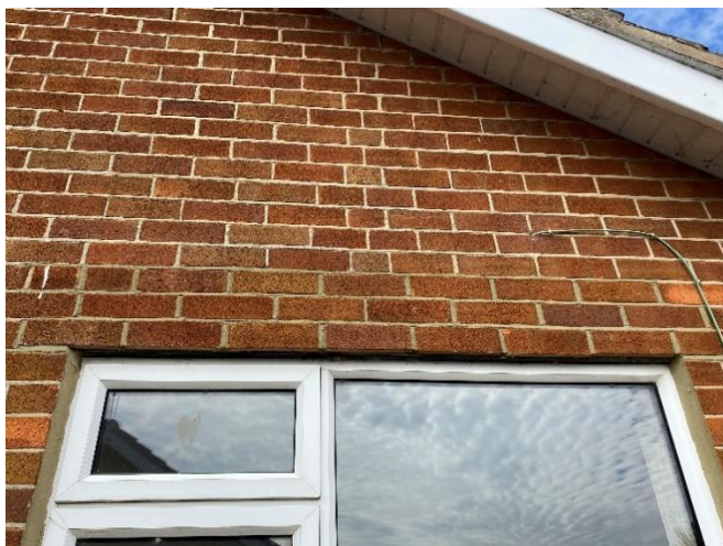
Photo 21: Brickwork and lintel (replaced) above the Rear Reception Room window
