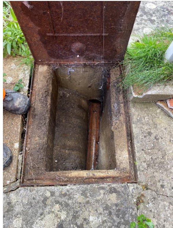
Photo 12: Inspection chamber adjacent to the Southeast corner of the main property
