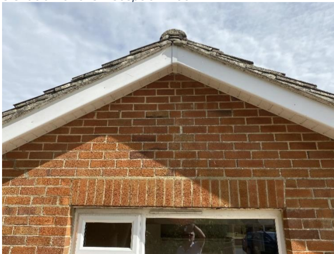
Photo 7: Repointing to the wall above the Front Bedroom window
