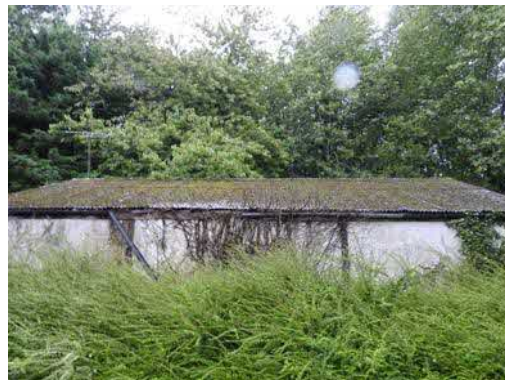
Fig. 5 Ridge and roof panels
