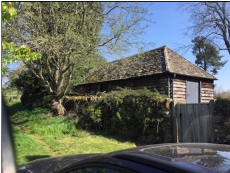
Figure 20: View of the outbuilding from Water Lane
