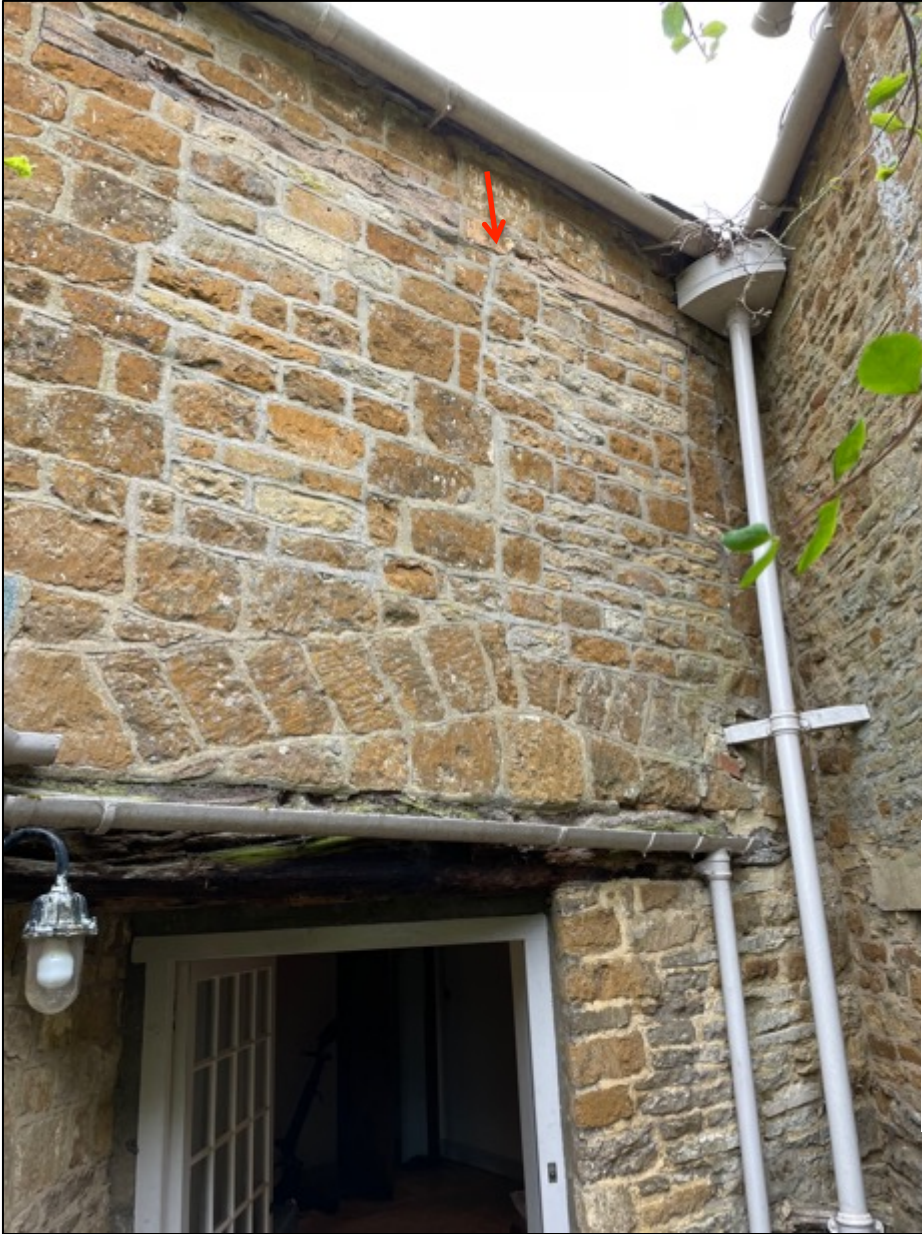
Figure 12: Left, blocked opening of what appears to be possibly a single opening externally, but as two openings internally (right).
