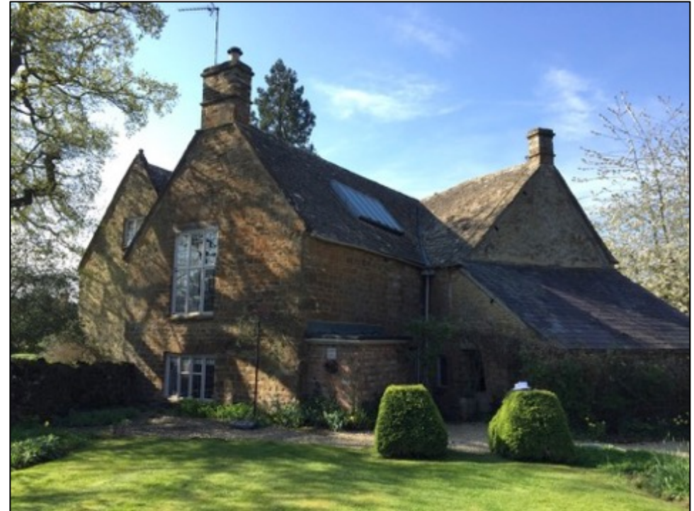
Figure 4: Northwest corner of the west range, garage/lean-to and roof of the northwest range.
