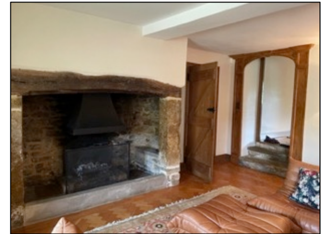
Figure 29: G2 – Inglenook fireplace, and doorways into G1 and G4
