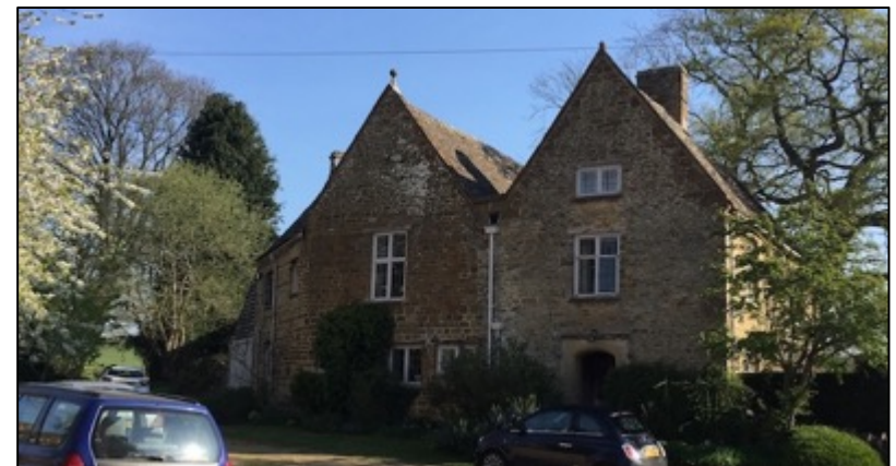
Figure 14: Top – historic photograph, date unknown, presumably pre-1900 before the stairs were inserted into G1 and the front door moved to G1: east range from west range. Right – photograph shows moved door and the window of the former door.
