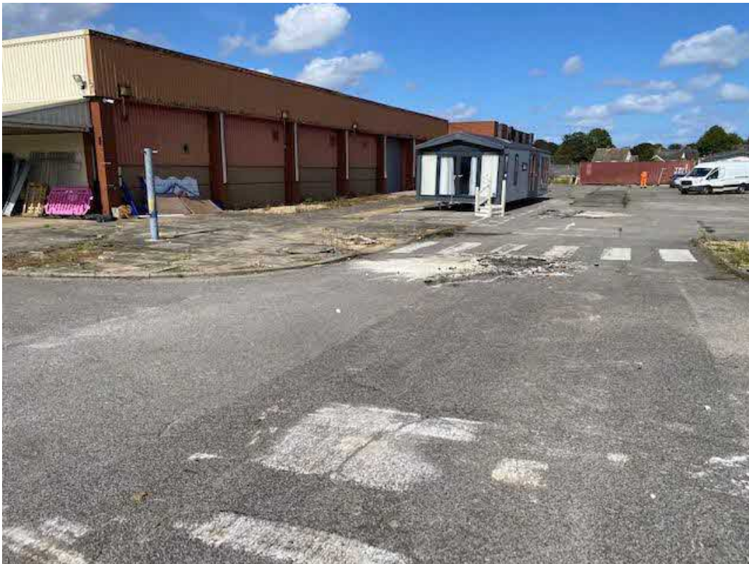
Photograph 2 – North west facing view of the site.
