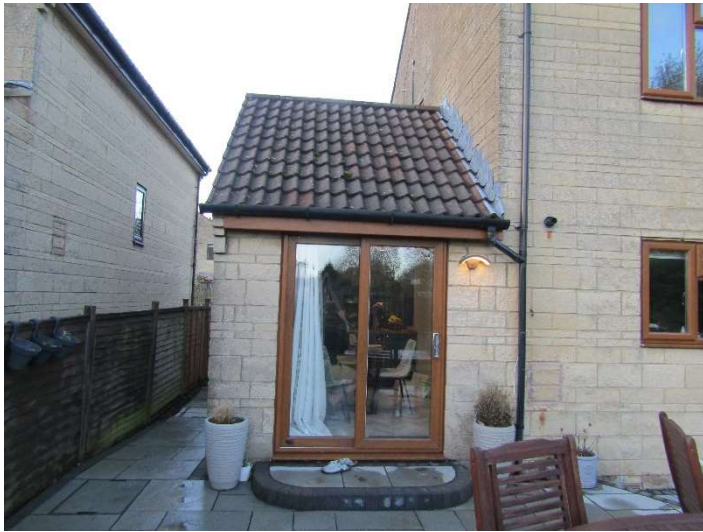
Rear of side extension to garage
