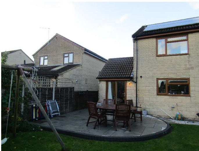
Rear extension showing single storey to be built above and adjoining property
