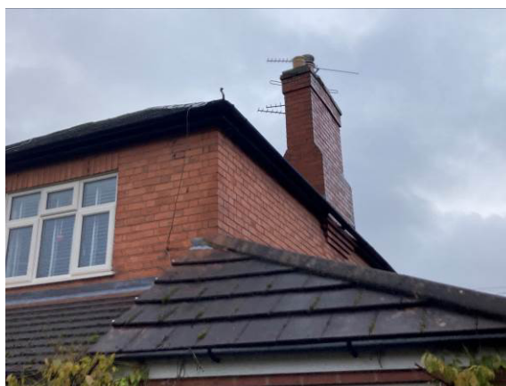
Rear junction of house and garage
