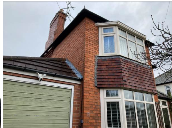
Front (west face) of house and garage
