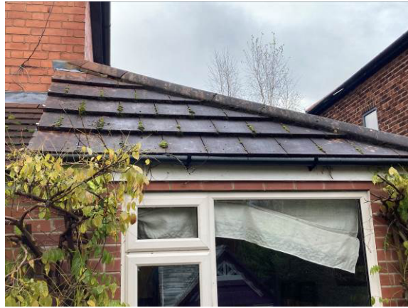
Garage extension (rear)
