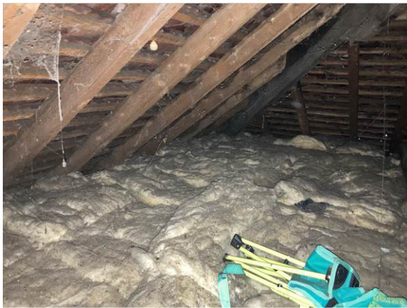
Loft interior man house
