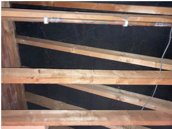
Underside of garage roof
