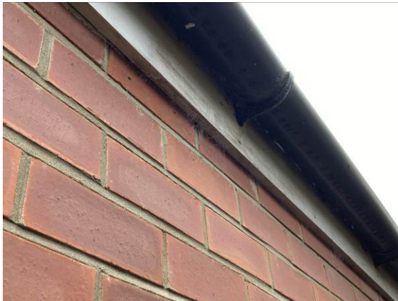
Close up of sealed roof edge
