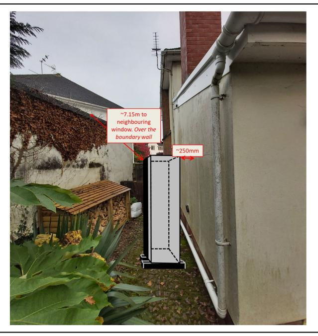
Client: 23-10-14 John Davies Address: 4 South Rise, Cardiff, CF14 0RH Project: Vaillant aroTHERM plus 10kW ASHP Detail: ASHP elevation plan view
