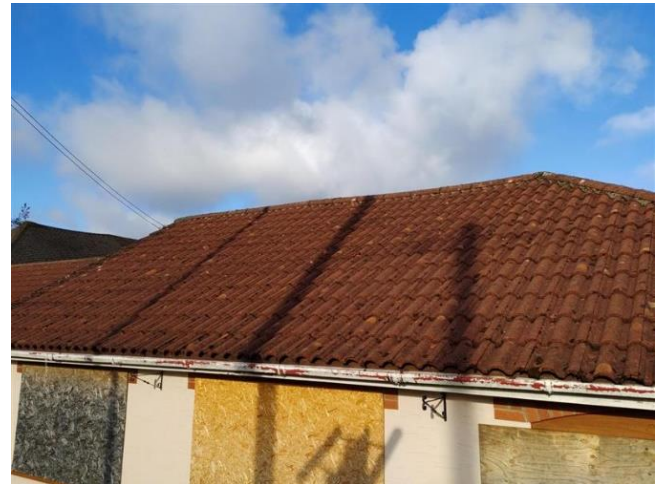
Figure 8 – View of the roof and southern aspect of the building.
