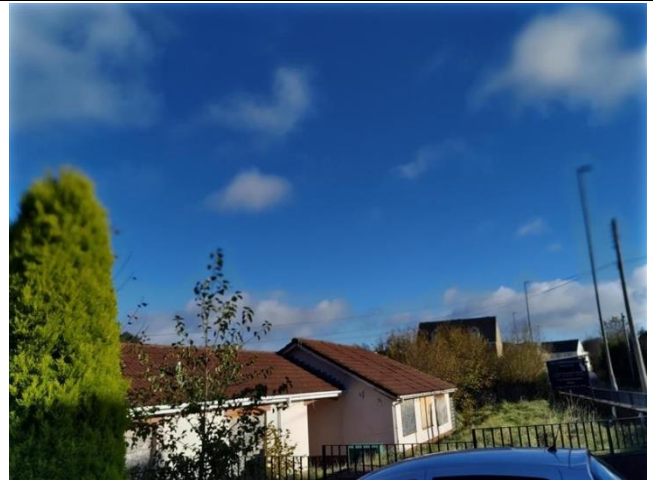
Figure 2 – View of the onsite building, looking east.
