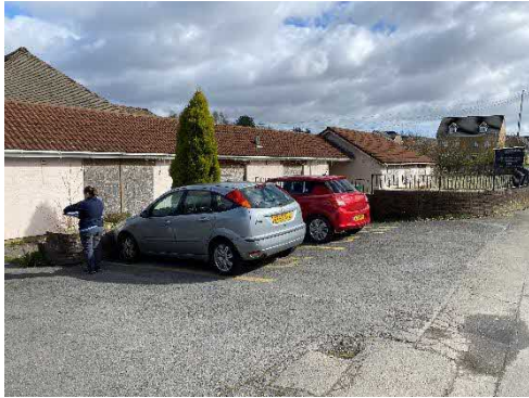
Figure 5 – Southern aspect of the building.
