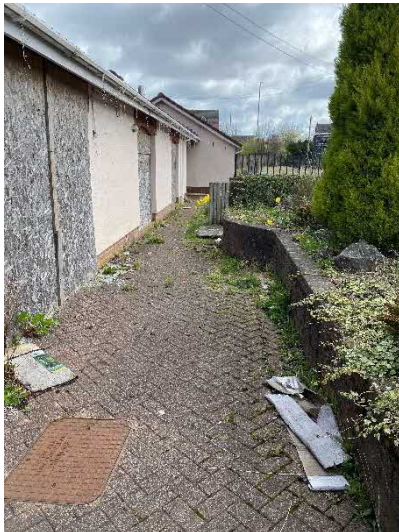
Figure 7 - Southern aspect of the building, looking east.
