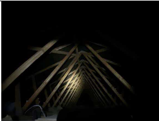
Figure 13 - Loft space at the east of building.
