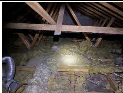
Figure 10 – Loft space at the east of the building.
