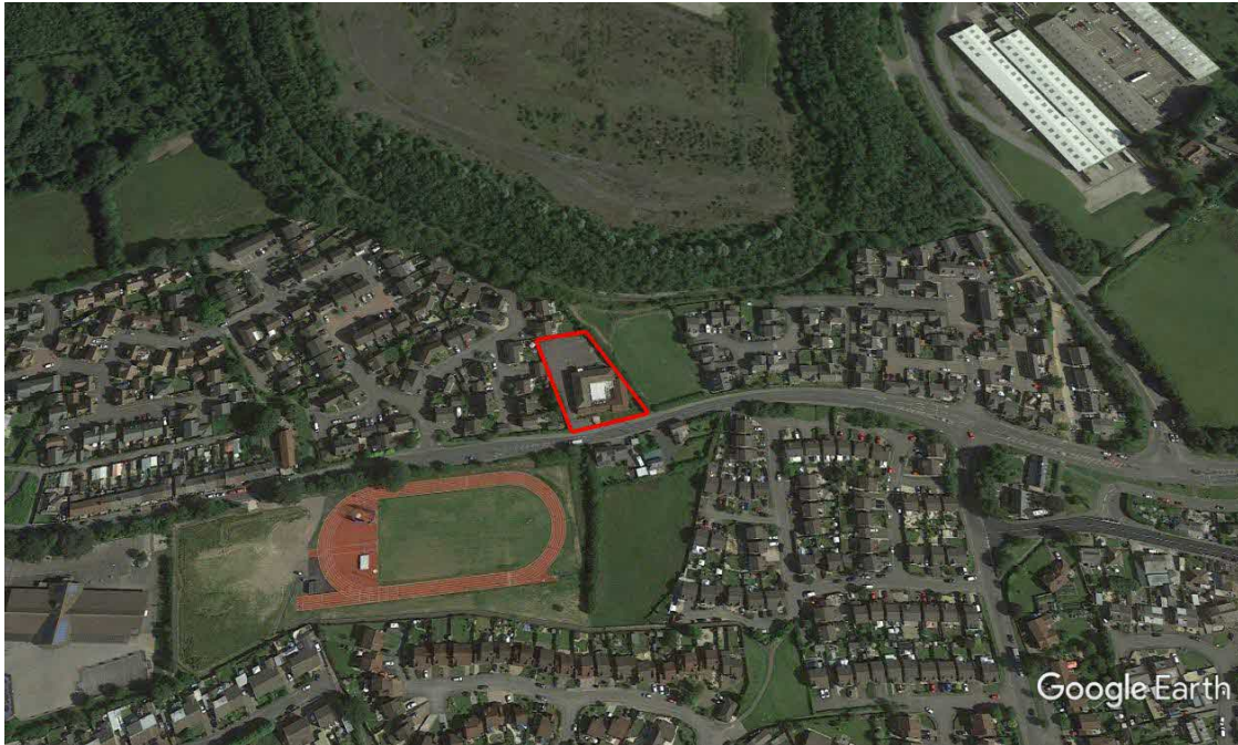
Figure 2 - Aerial Image of the wider site (red line shows the site boundary Image used under licence (©2022 Google). Imagery date 20/07/2021.
