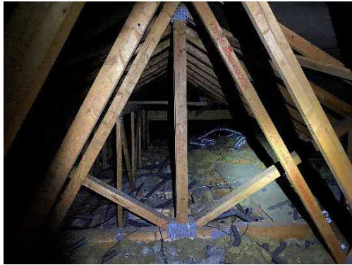
Figure 11 - Loft space at the east of the building.
